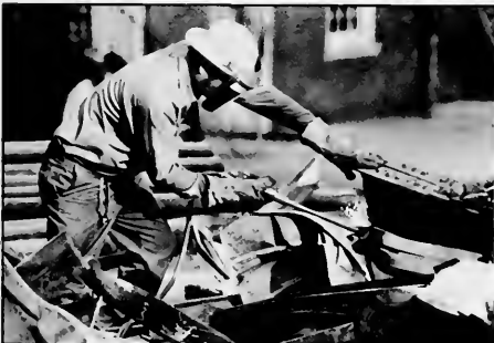
The Can being torn down. 8/77
