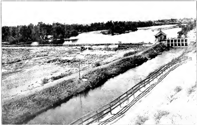
Yukone River and Intake, Sunnyside Canal
