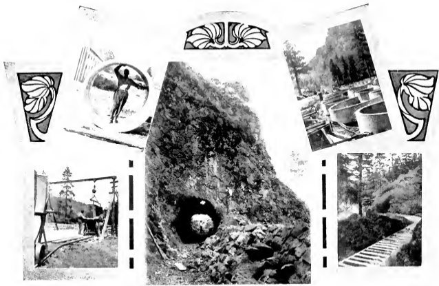
Construction Work on the Teton Canal.
