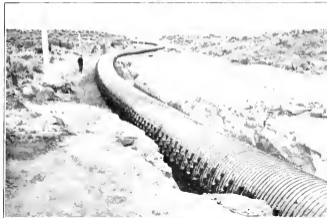
Stave Pipe Construction on Mabton Canal
