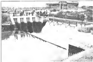
Weir at Head of Zillah Spillway
