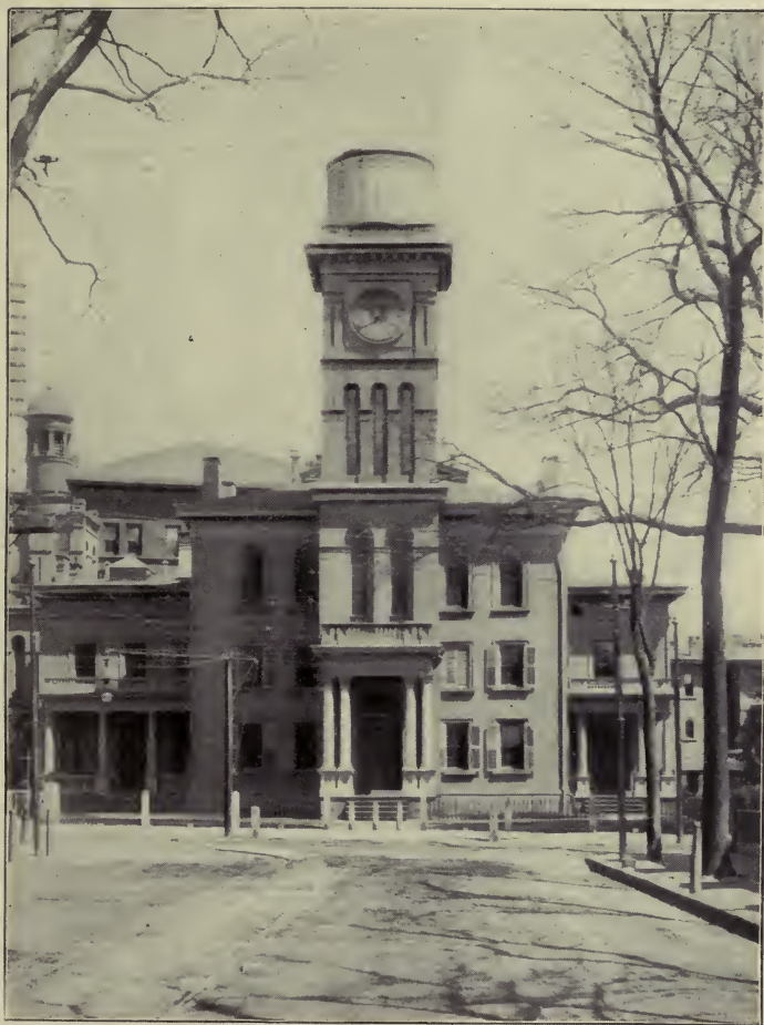
SOUTH SHEFFIELD HALL
