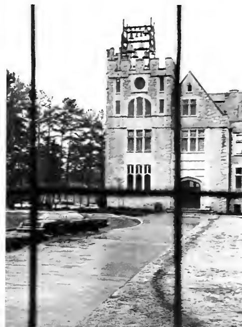
While the carillon bells ring out and the rain falls, stately Lupton Hall stands proudly overlooking the main quadrangle.
