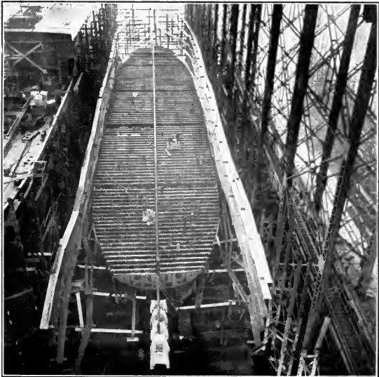
THE SHIP THAT WAS BUILT IN TWENTY-SEVEN DAYS View of the Tuckahoe on the third day, showing floors in place.
