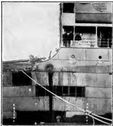
CUTTING A LAKE SHIP IN TWO PREPARATORY TO TAKING IT TO SALT WATER
