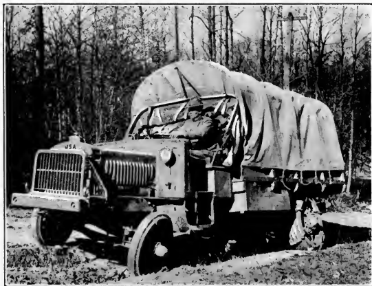
THE "LIBERTY" TRUCK, DESIGNED BY ARMY ENGINEERS
