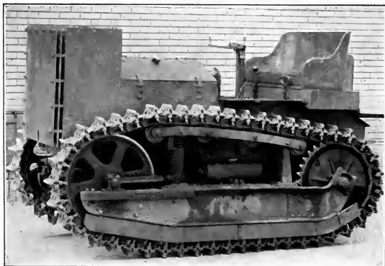
LIGHT CATERPILLAR TRACTOR FOR HAULING 3-INCH GUN
