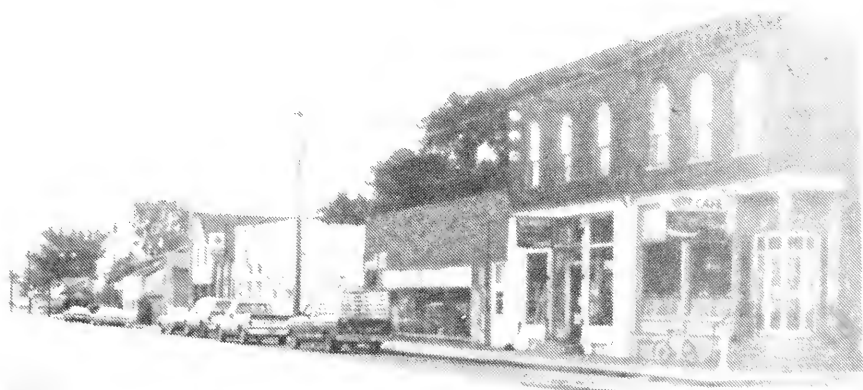
East corner of Main and Union Streets on the north side
