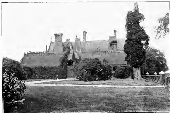
GAWDY HALL --SOUTH SIDE.
