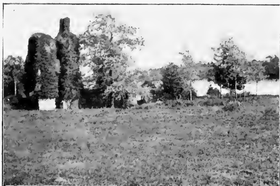
OLD MANOR HOUSE, BOULSTON - WEST END.
