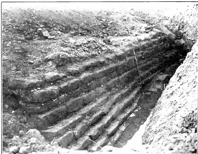
Fig. 13. - The dwelling-house : offsets at north corner.
