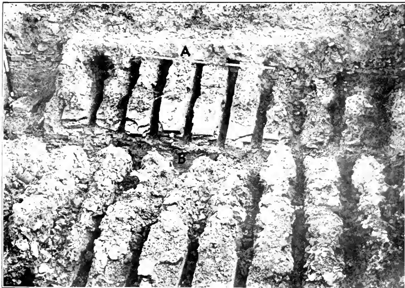
Fig. 17.—The double flue kiln: interior of kiln. Cross-flue walls with springers of arches still in position. A, remains of oven-floor; B, right-hand main flue. The survey pole stands in the rear right-hand corner of the kiln.
