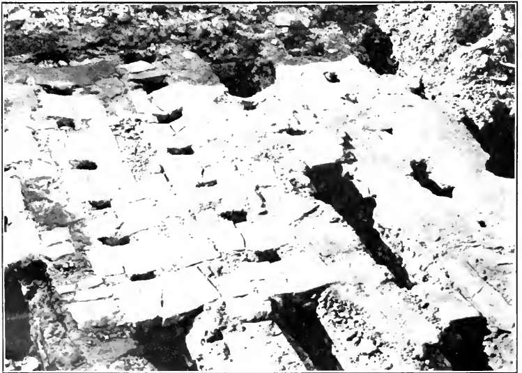
Fig. 29. No. 5 tile kiln: view of oven-floor partly stripped, showing tiles used to bridge cross-flues. Note V-ended brick used to repair floor.
