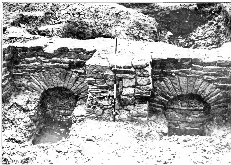
Fig. 16.—The double flue kiln: front view of main arches, showing tile fillings.
