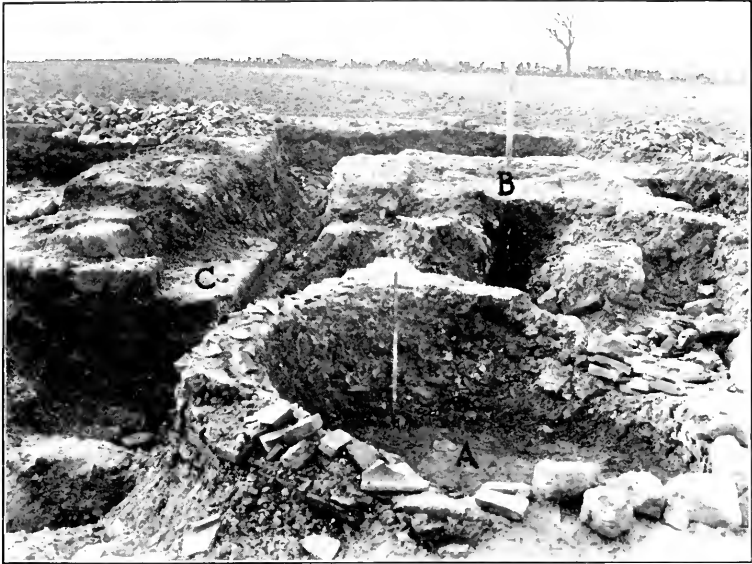
Fig. 26. --Part of the main kiln-plant. A, floor and superstructure of round pottery kiln ; B, the ruined No. 2 pottery kiln ; C, the outer casing of No. 3 tile-kiln, with oven floor beyond.
