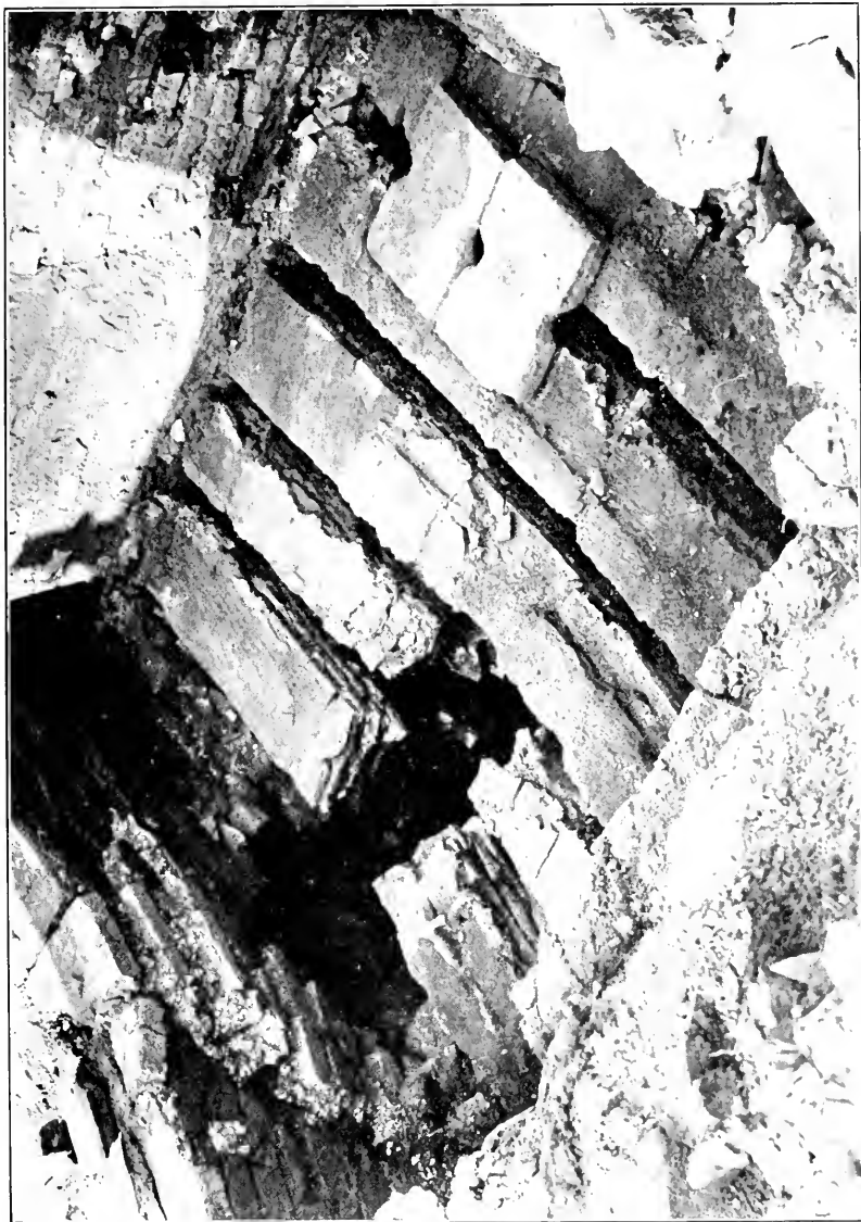
Fig. 22. No. 1 pottery kiln. First stage in building oven-floor, showing cross-walls and flues, and arch of main flue, with two notched tiles in position. To face p. 34
