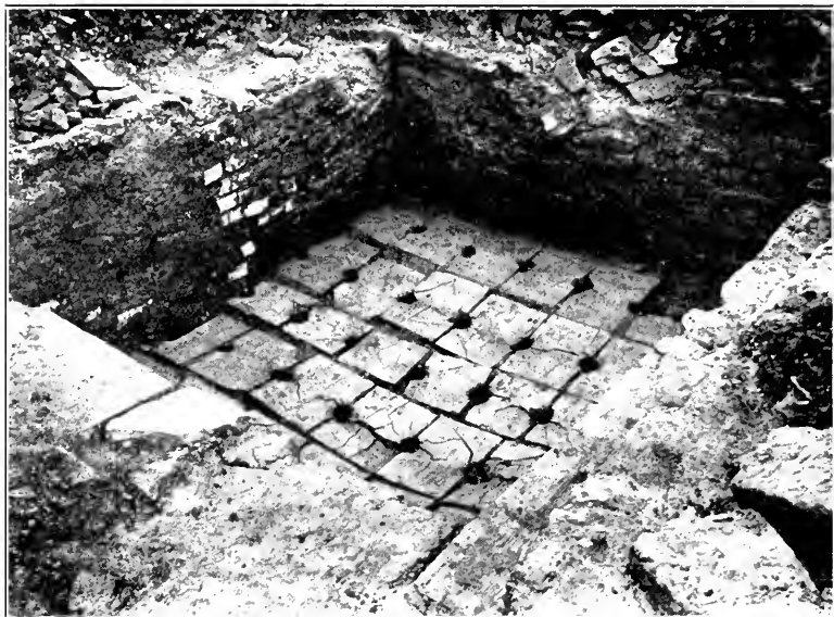
Fig. 23. No. 1 pottery kiln. Second stage in building oven floor, showing all tiles in position and partly daubed.
