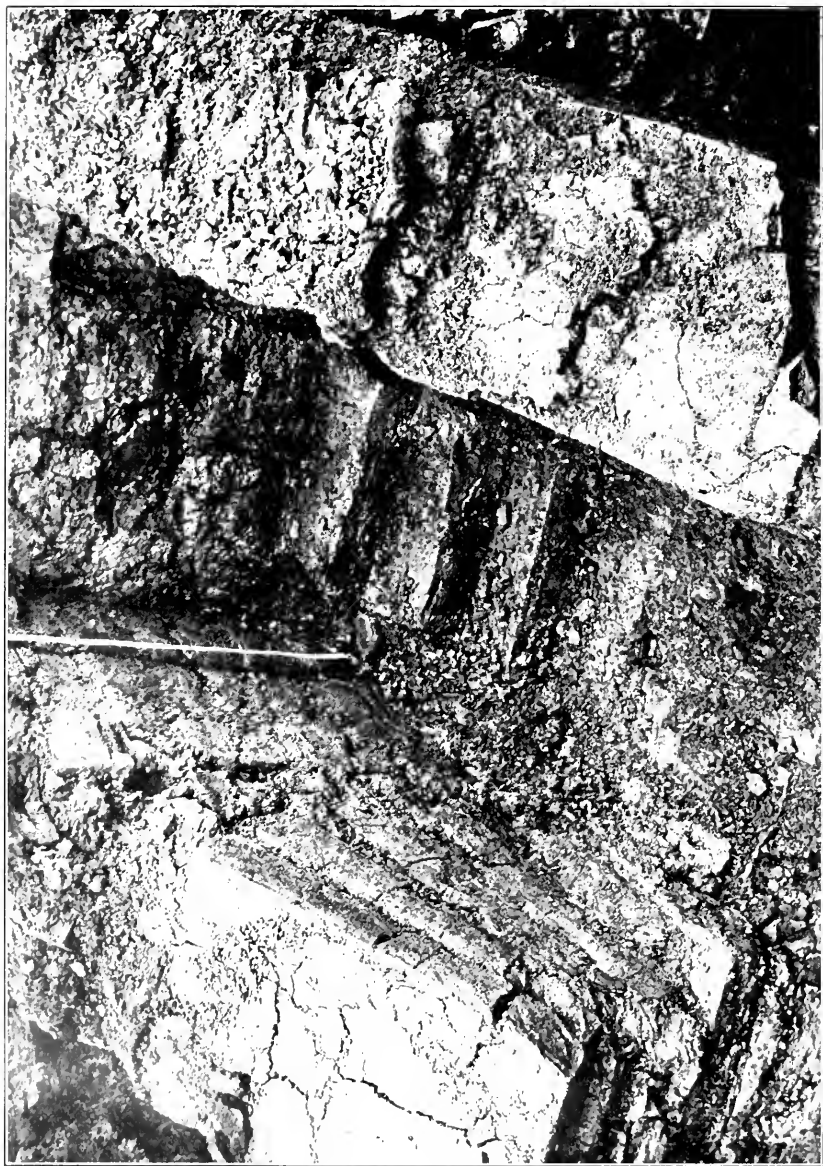
Fig. 18.—The double-flue kiln. Detail of cross-flue wall, showing the gap between tiles and arch filled in with daub, and stepping of brickwork. To face p. 27.
