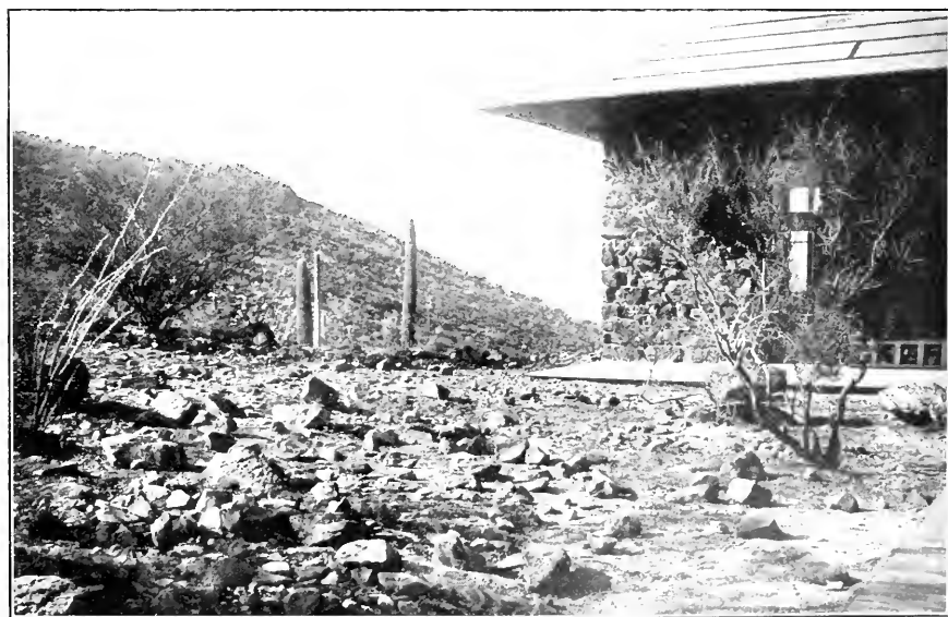
DESERT BOTANICAL LABORATORY. VIEW IN REAR OF THE BUILDING, LOOKING SOUTHWESTWARD.
