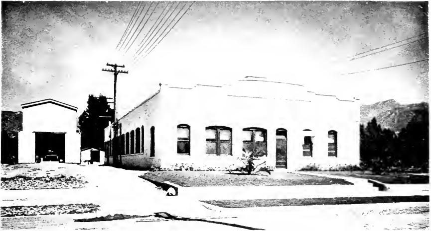
PASADENA OFFICE AND ERECTING BUILDING.
