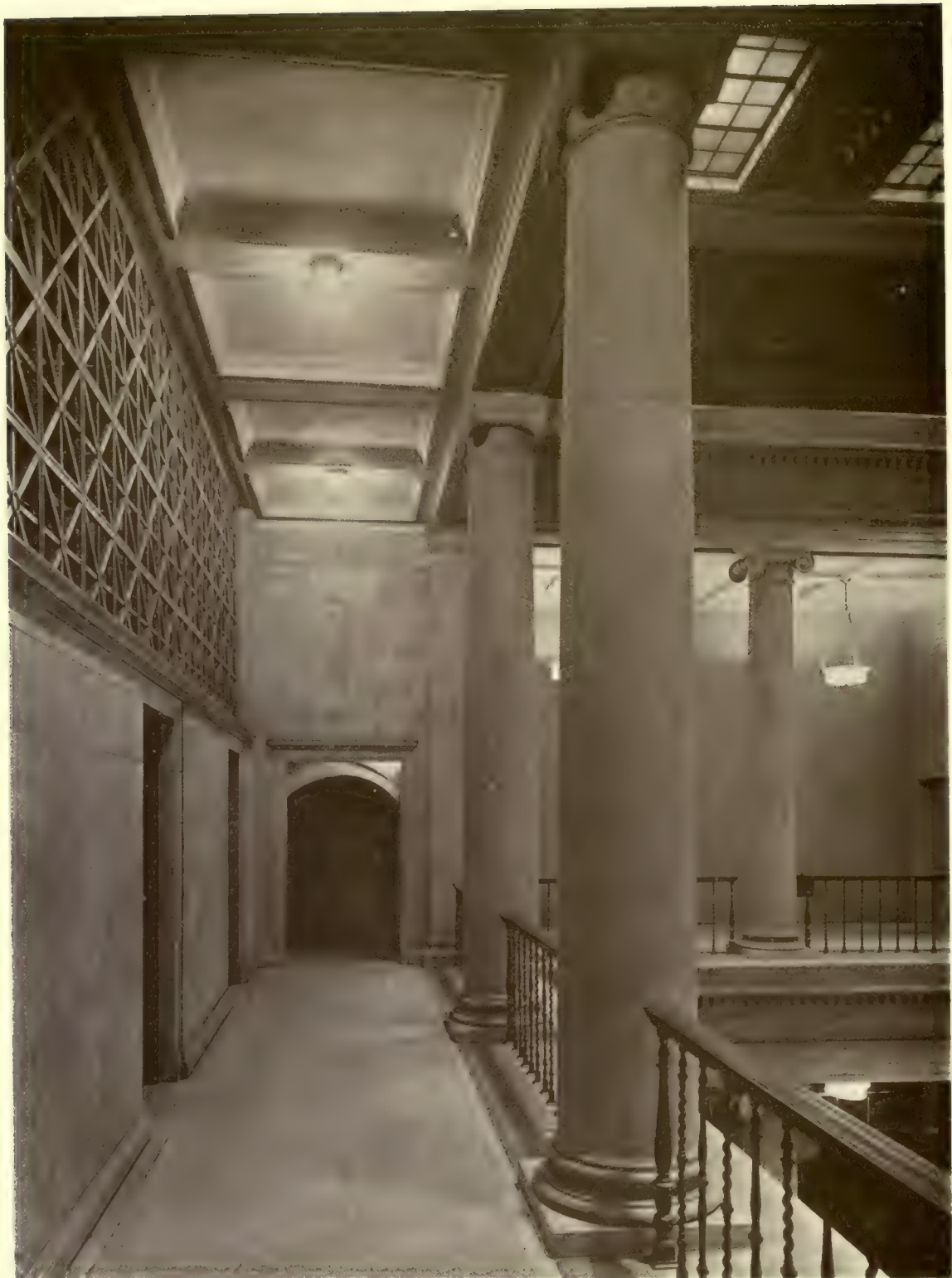
NORTH GALLERY OF BOOK ROOM, JOS. J. HILL REFERENCE LIBRARY, ST. PAUL, MINN. ELECTUS D. LITCHFIELD, Architect, New York
