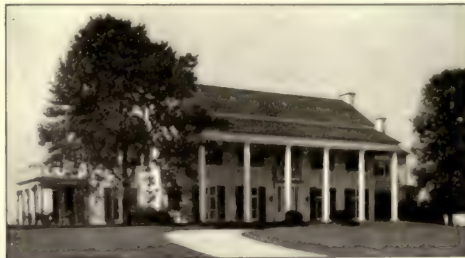
Shingled Walls and Brick Chimneys finished with Cabot's Old Virginia White. John Russell Pope, Architect, New York
