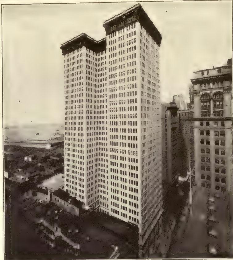
ADAMS BUILDING, NEW YORK CITY Structural steel furnished through Post & McCord, Inc. Francis H. Kimball, Architect
