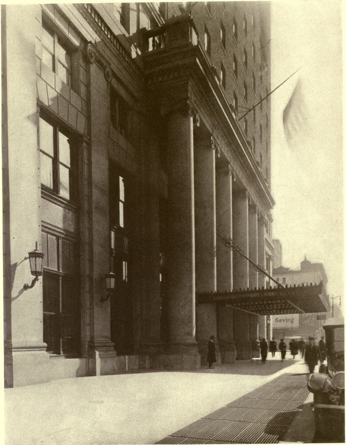
HOTEL PENNSYLVANIA MCKIM, MEAD & WHITE, Architects, New York
