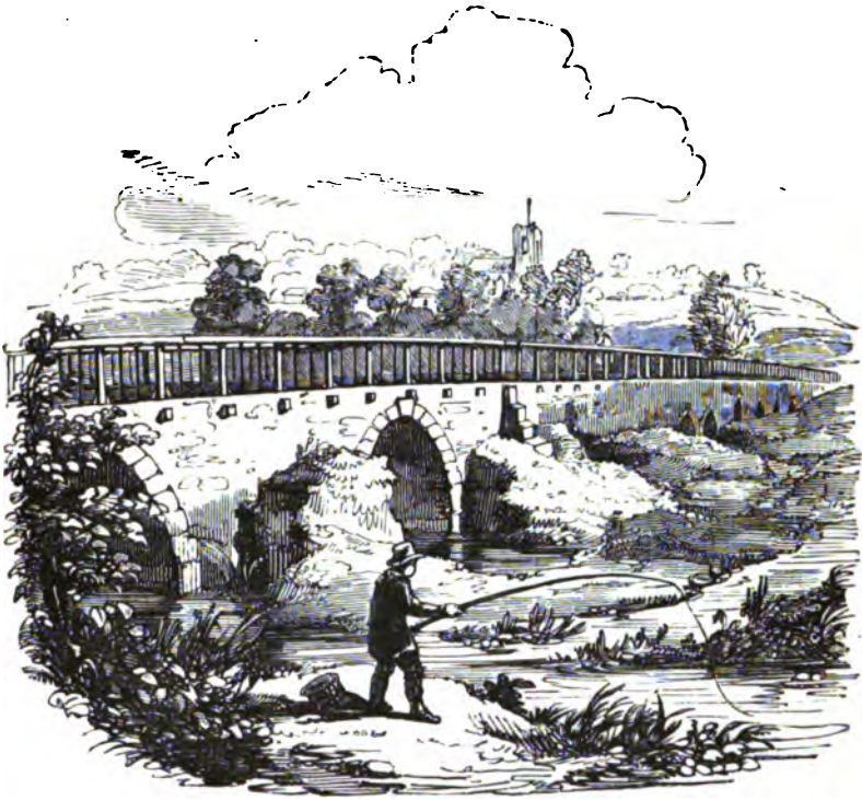
OLNEY BRIDGE, BUCKINGHAMSHIRE.
