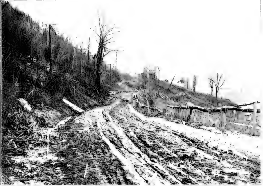
FIG. 1.—TYPE OF ROAD IN MASSACHUSETTS BEFORE IMPROVEMENT.
