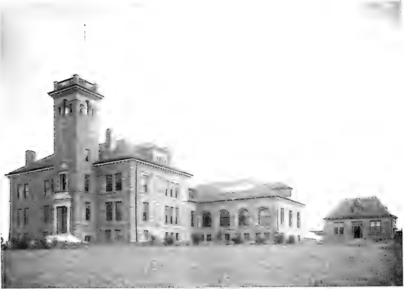
FIG. 1.—ADMINISTRATION AND LABORATORY BUILDING OF OHIO STATION.
