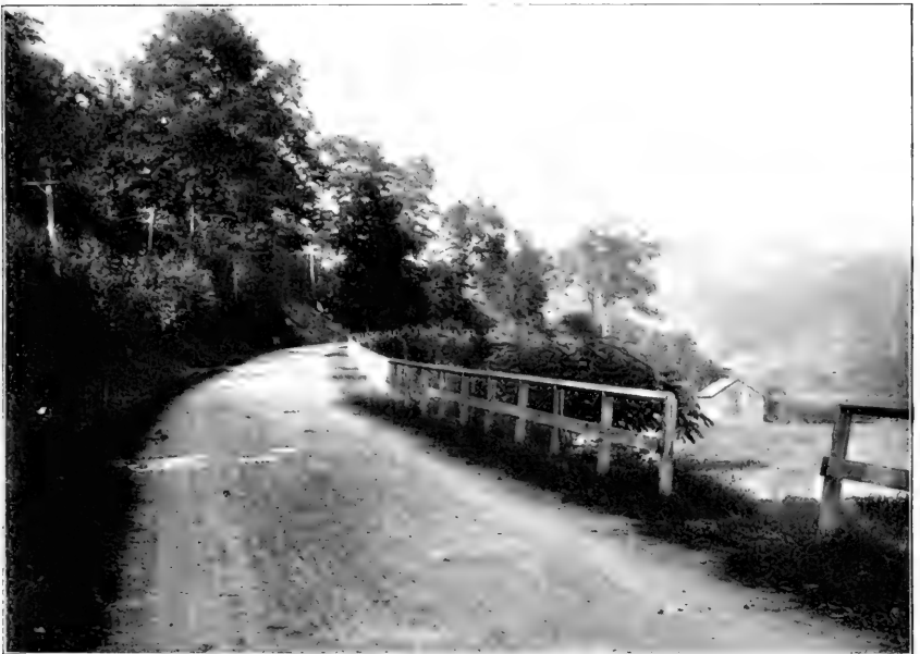
FIG. 2.—TYPE OF ROAD IN MASSACHUSETTS AFTER IMPROVEMENT.
