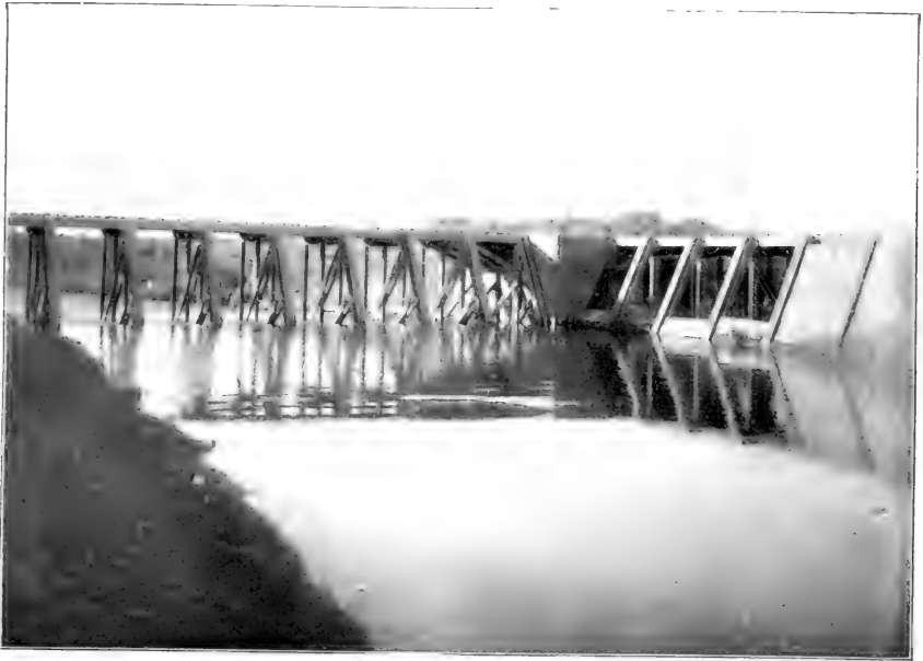
FIG. 1.—A CHECK AND LATERAL GATE ON MAIN CANAL.
