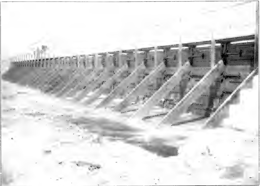
FIG. 1. CANAL WASTE GATE CLOSED.
