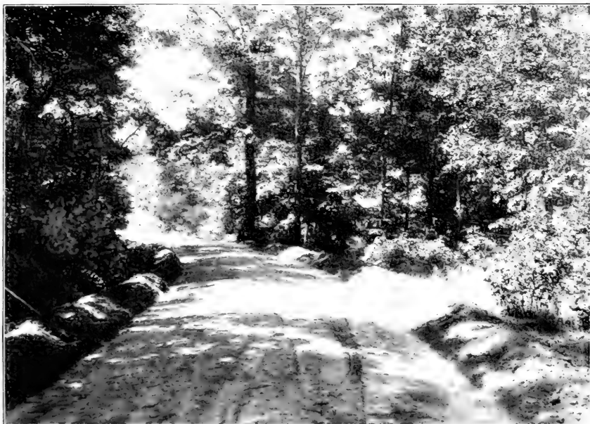
FIG. 1.—THE ROLLED FOUNDATION OF AN OBJECT-LESSON ROAD BUILT AT HOT SPRINGS, VA., UNDER THE AUSPICES OF THE OFFICE OF PUBLIC ROAD INQUIRIES OF THE DEPARTMENT OF AGRICULTURE.
