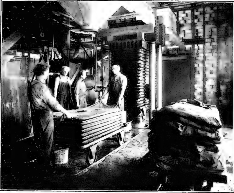
FIG. 1.—PRESSING OLIVES (BACK); STRIPPING THE CAKE (FRONT).
