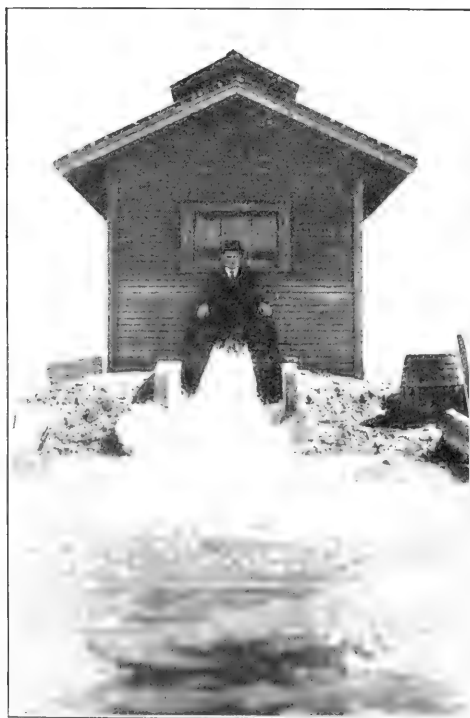
FIG. 2.—ONE OF TWENTY-TWO PUMPS USED FOR IRRIGATING ALFALFA AT DEMING, N. MEX.
