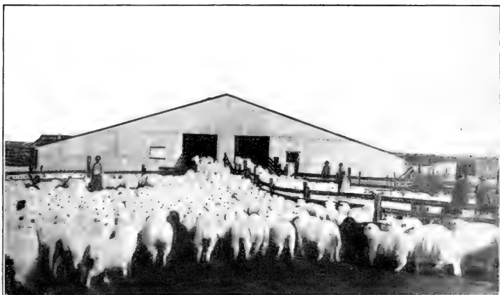
FIG. 1.—SHEEP ENTERING SWEATING PENS OF A REMODELED SHEARING SHED AT BITTER CREEK, WYO.
