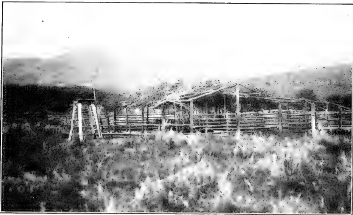
FIG. 1.—TYPE OF SHELTER FREQUENTLY USED FOR SHEARING SHEEP ON WESTERN RANGES.
