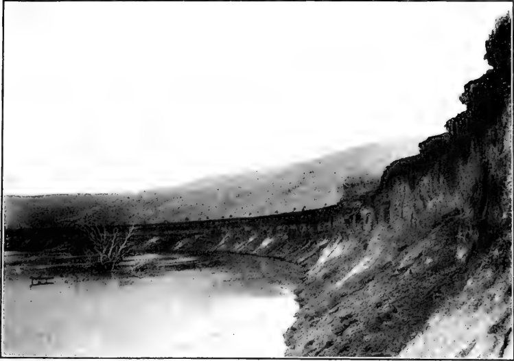
FIG. 1.—AN UNPROTECTED RIVER BANK.
