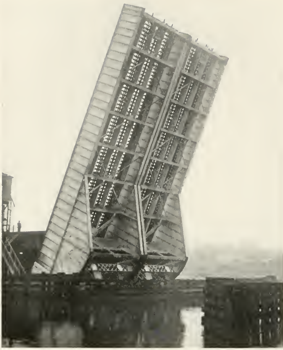
NEW ROLLING LIFT BRIDGE
