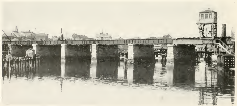
RAILROAD BRIDGE ACROSS HARBOR
