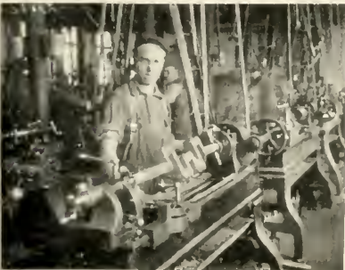
FINISHING A CRANK SHAFT
