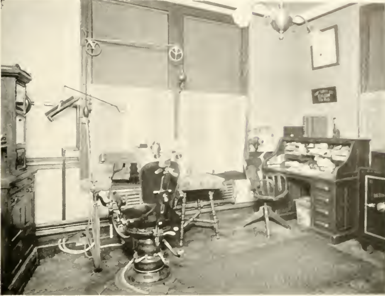
One of the Operating Rooms—Notice Up-to-date Equipment
