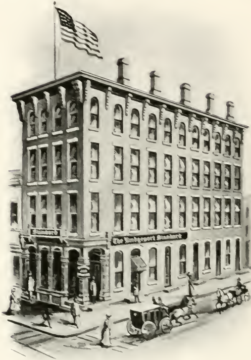
The Standard Office, cor. Fairfield Ave. and Middle St.
