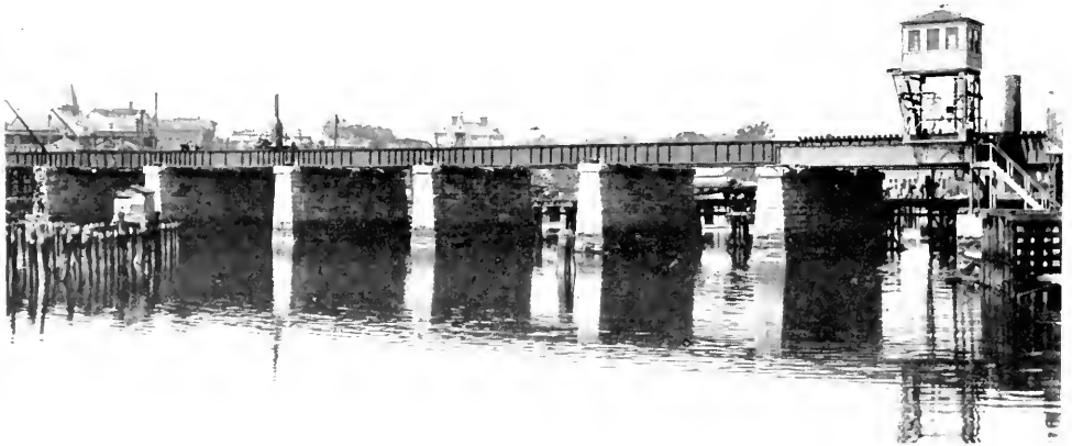
RAILROAD BRIDGE ACROSS HARBOR
