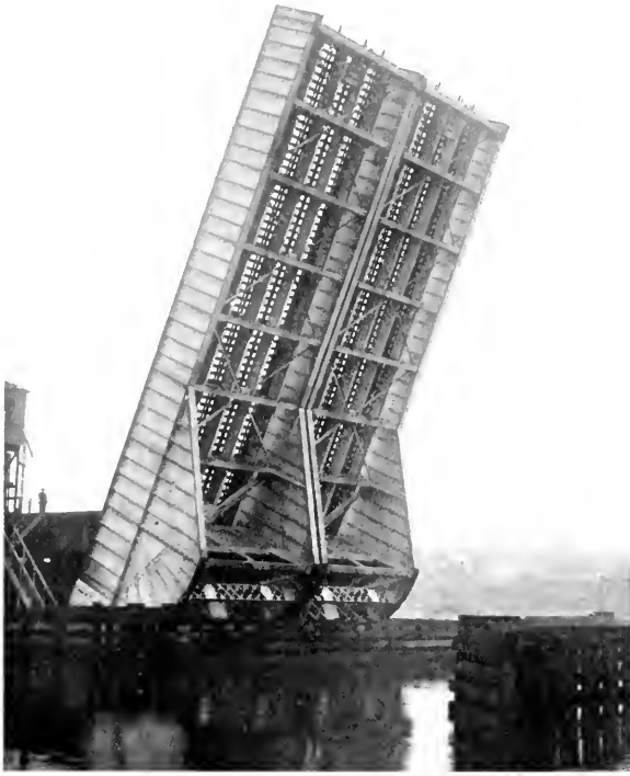
NEW ROLLING LIFT BRIDGE
