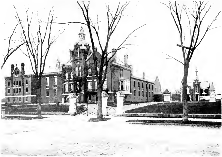
FAIRFIELD COUNTY JAIL
