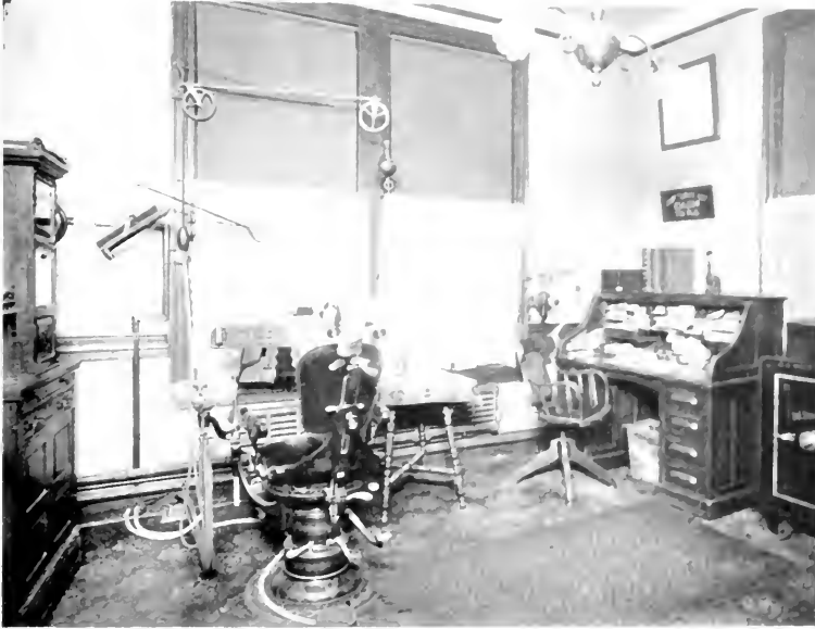
One of the Operating Rooms. Notice Up-to-date Equipment.
