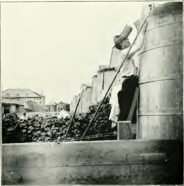
FIG. 48.—The Screening Gang at work securing the Cisterns. New Orleans, 1905.
