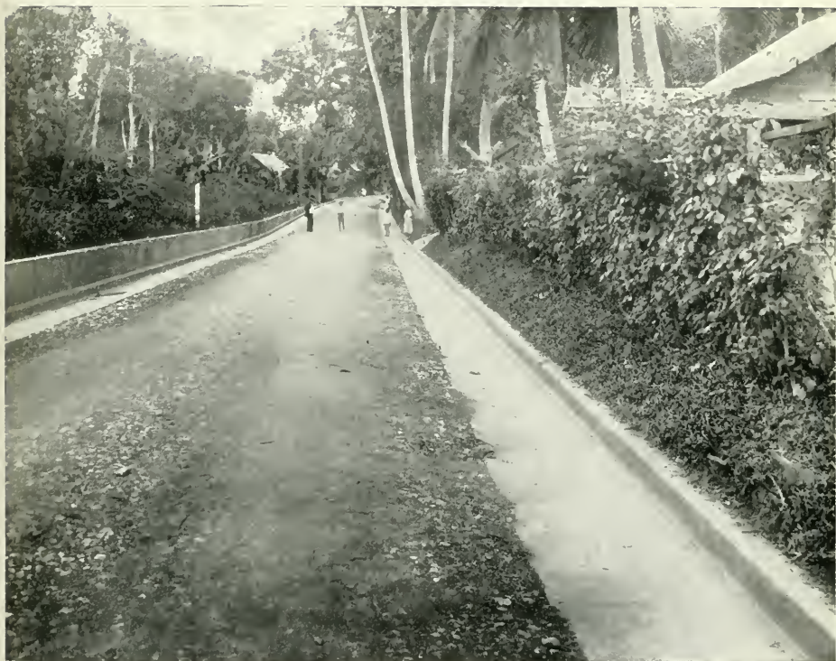
FIG. 57.—A Road in Port of Spain, properly graded, with well-made concrete side drains.
