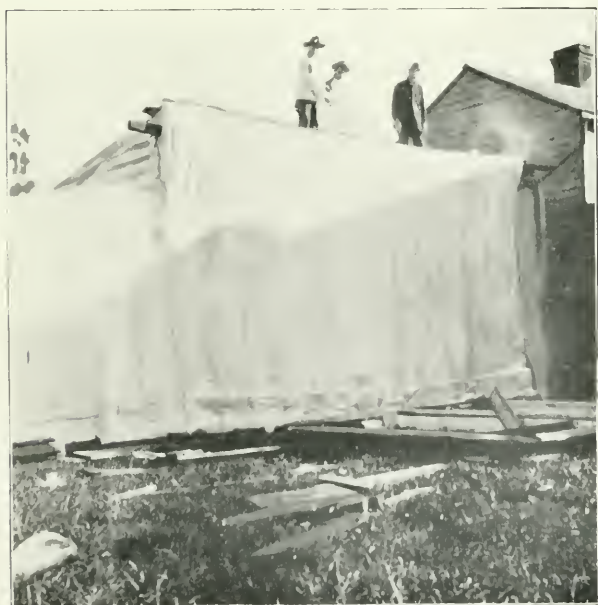
FIG. 53.—A Carefully-papered Outhouse, ready for Fumigation. New Orleans, 1905.
