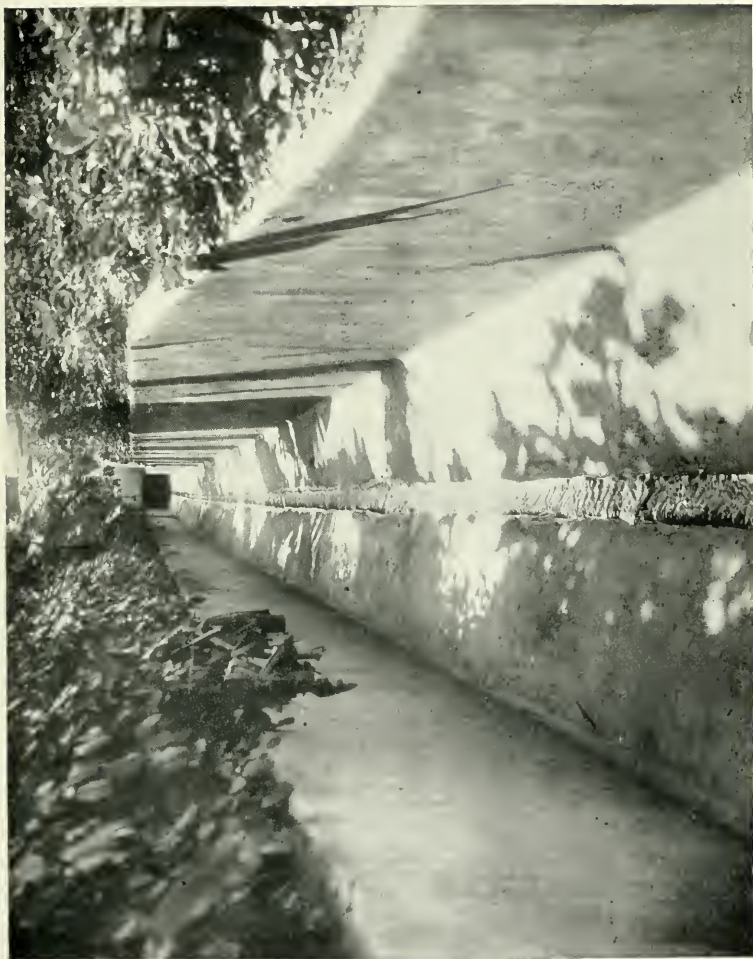
FIG. 3.—The Bed of a Water-course, made in concrete, to prevent the formation of puddles and the breeding of mosquitos. Trinidad, 1909. (From Mosquito or Man? )
