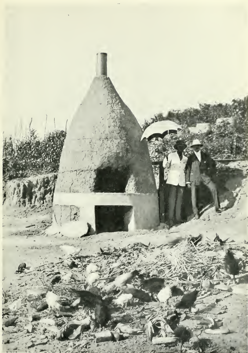
FIG. 58.—The "Bee Hive Destructor." A very simple, efficient, and cheap form of destructor, constructed out of "swish." Secondee, Gold Coast.
