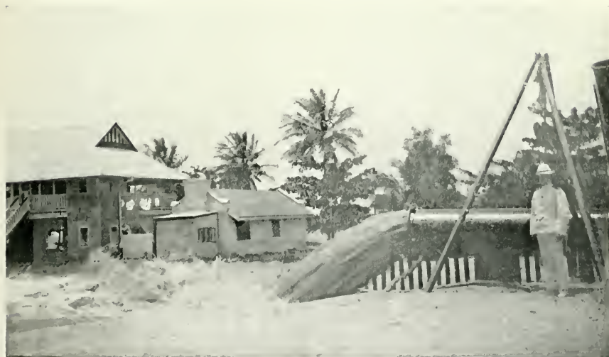
FIG. 50.—Modern Method of filling in a Swamp by means of a powerful Sand Pump. Lagos, 1910.
