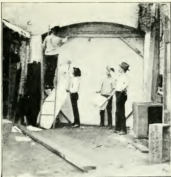
FIG. 52.—The Papering Gang at work, rendering rooms tight before Fumigation. New Orleans, 1905.
