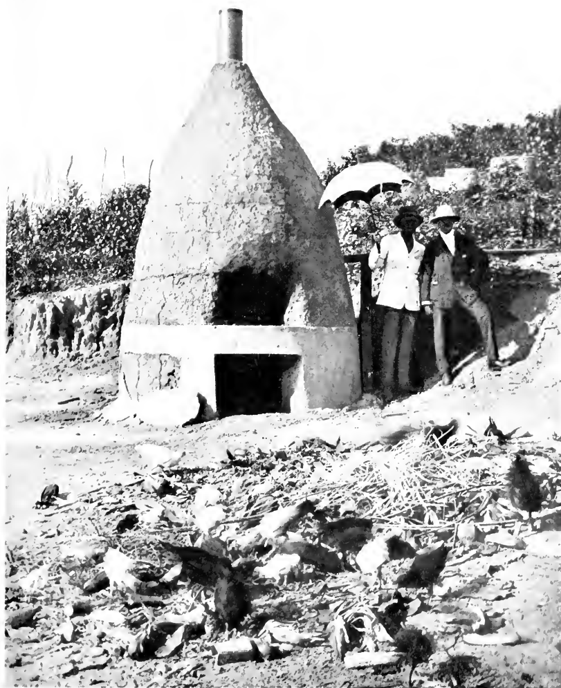
FIG. 58.—The "Bee Hive Destructor." A very simple, efficient, and cheap form of destructor, constructed out of "swish." Secondee, Gold Coast.
