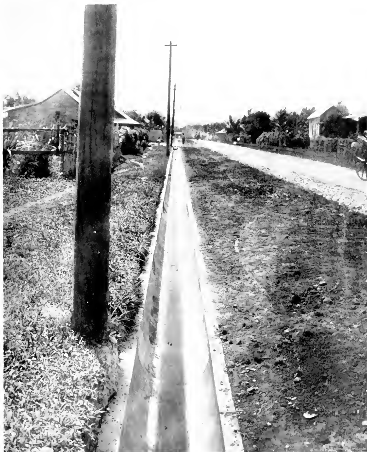
FIG. 4. —A Concrete Roadside Drain, Port of Spain, Trinidad.
