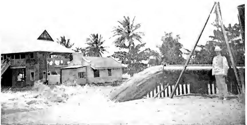
FIG. 50.—Modern Method of filling in a Swamp by means of a powerful Sand Pump. Lagos, 1910.
