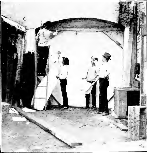
FIG. 52.—The Papering Gang at work, rendering rooms tight before Fumigation. New Orleans, 1905.
