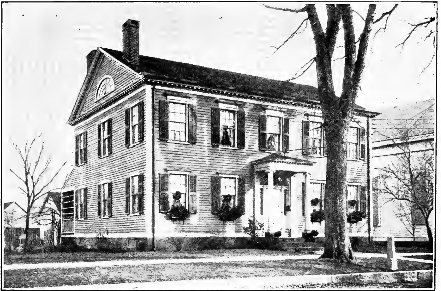
MAJOR LATHROP'S FOUR-CHIMNEY HOUSE MINUS TWO CHIMNEYS
