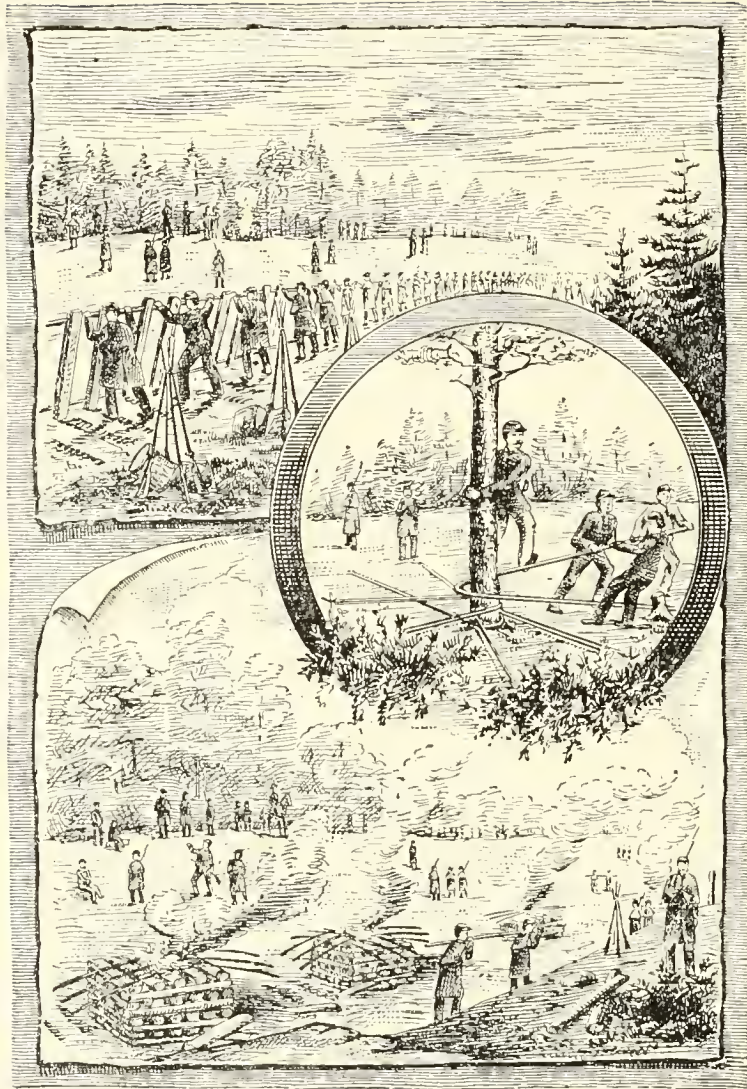
200th DESTROYING WELDON RAILROAD NEAR RICHMOND, VA.
