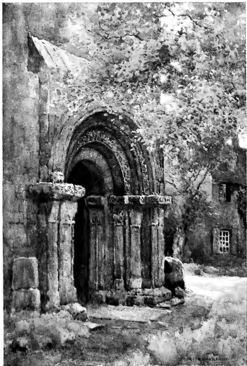
NORMAN PORCH, ST. LAWRENCE'S TOWER
