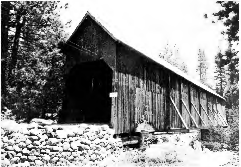
Covered bridge over South Fork of Merced River at Wawona
