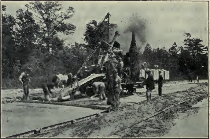
MODERN ROAD BUILDING
