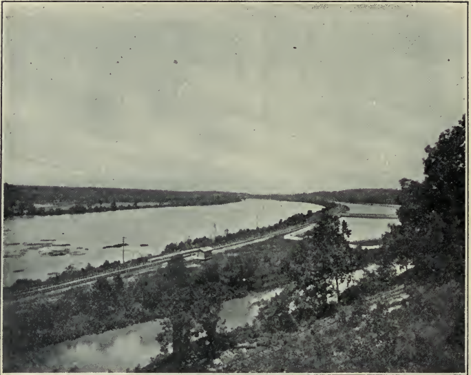
WATER SUPPLY FOR A CITY
