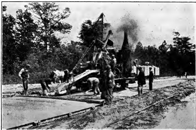
MODERN ROAD BUILDING
