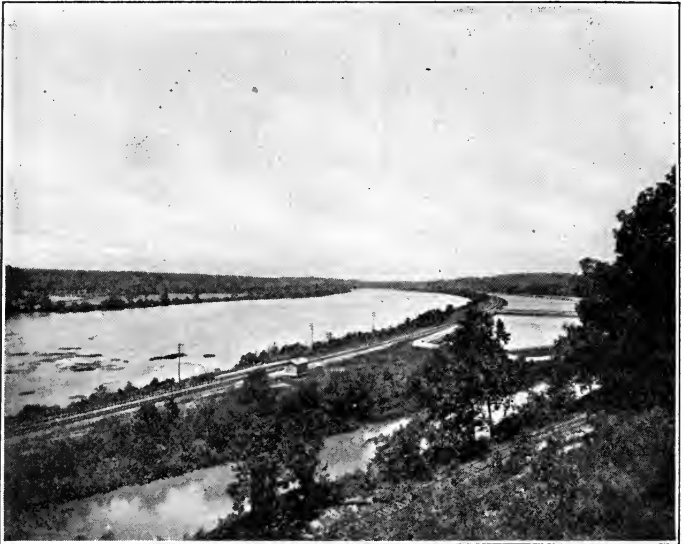
WATER SUPPLY FOR A CITY
