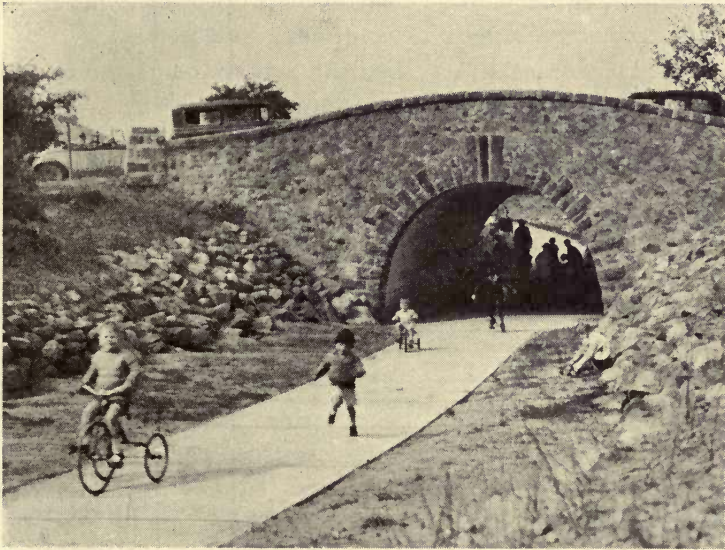
AN UNDERPASS GUARDS THE CHILDREN FROM MOTOR HAZARDS IN RADBURN, NEW JERSEY
