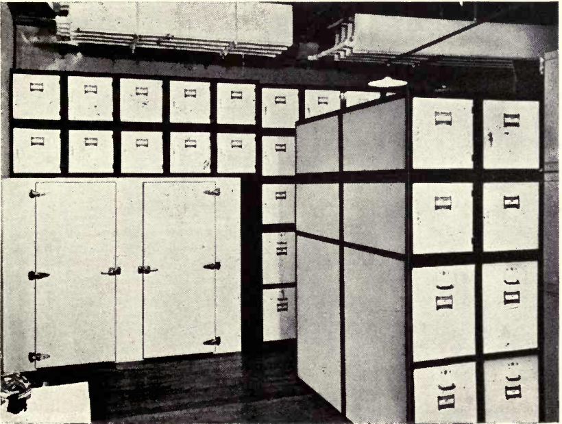
This arrangement makes the freezing cabinet easily accessible. Note that the lowest two tiers provide more space than top three tiers; they also bring more.
