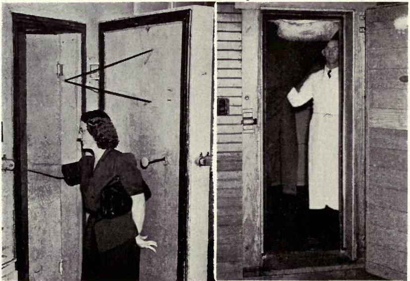
Exchange of air between the zero locker room and the warmer outside rooms is necessary. Here are two ways this has been managed by locker plant owners. Left, a double swinging door arrangement; and right, a heavy canvas curtain.
