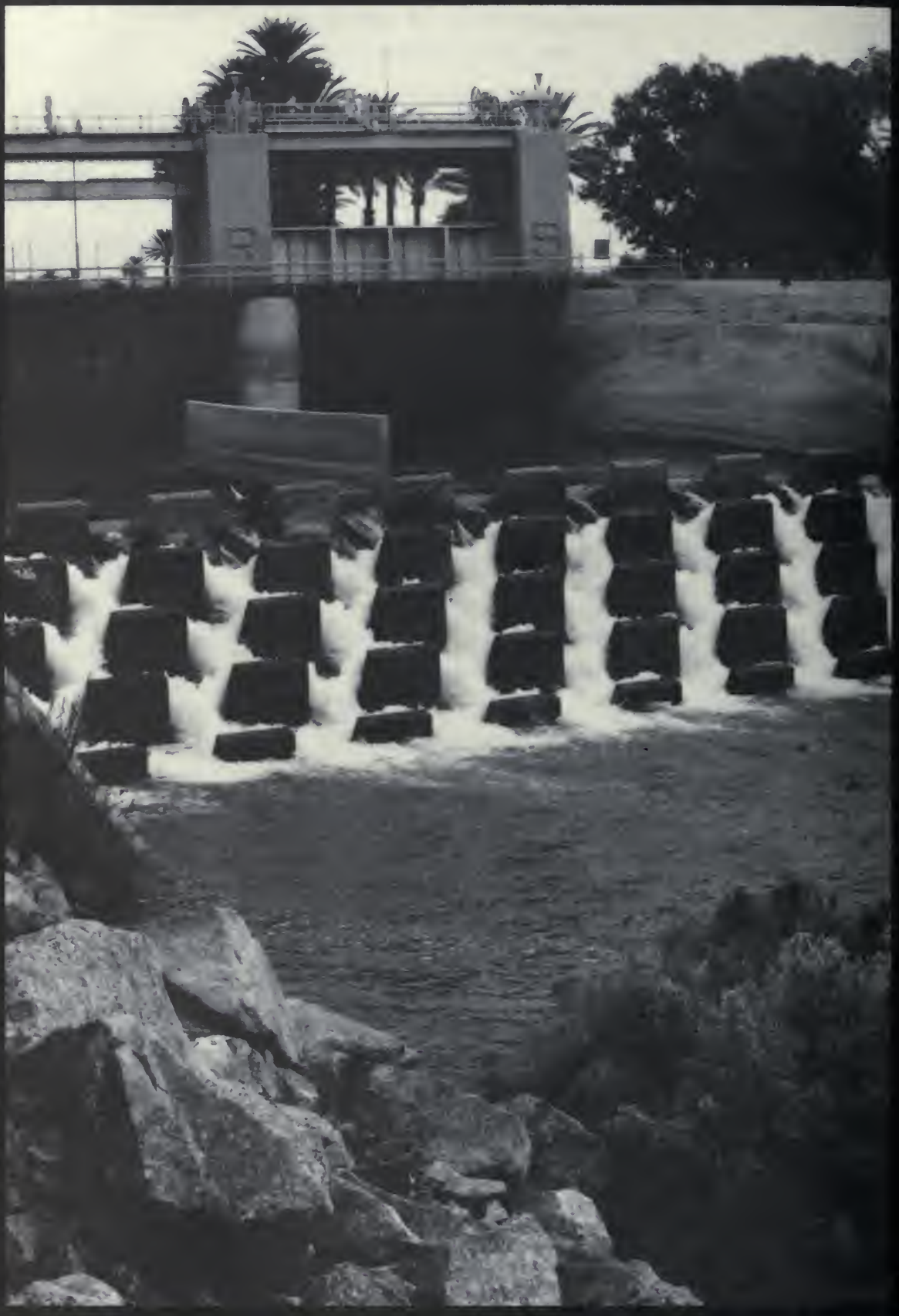
Control gates on the Colorado River Aqueduct.
