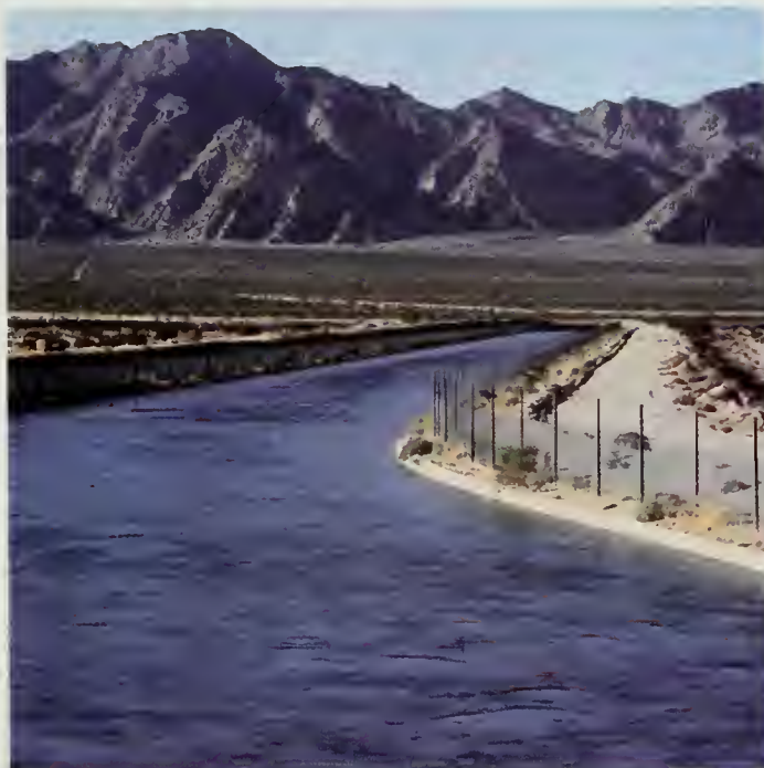
The Colorado River Aqueduct makes its way across the valley floor, with Iron Mountain providing the backdrop. This aqueduct has been providing about 1,000,000 af annually to the South Coast Region.
