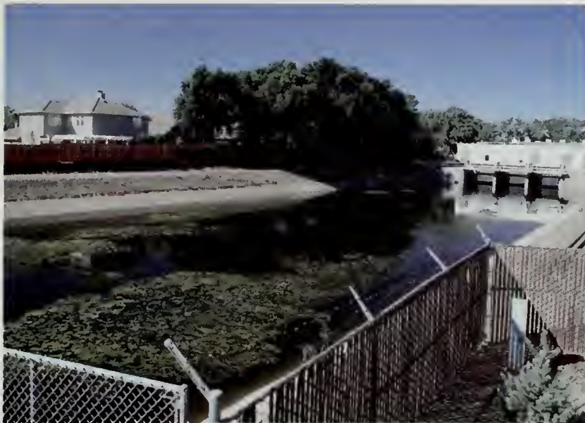
New housing construction in Sacramento County. Many new homes are being built in the flood plain. The pumps shown in the foreground pump rainfall runoff from the area into the Sacramento River during storms.
