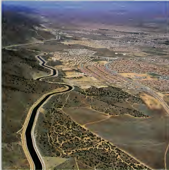
The East Branch of the State Water Project winds across sparsely vegetated hillsides past recently developed urban areas in the distance. Urban growth in the high desert area is expected to continue its rapid pace.
