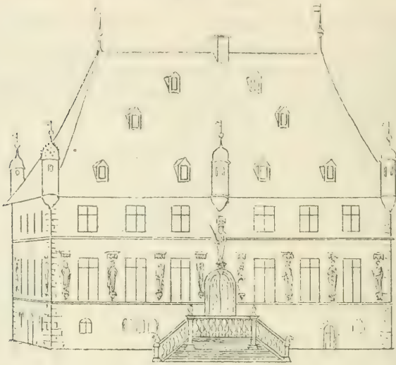
Das Rathhaus in Osnabrück.
