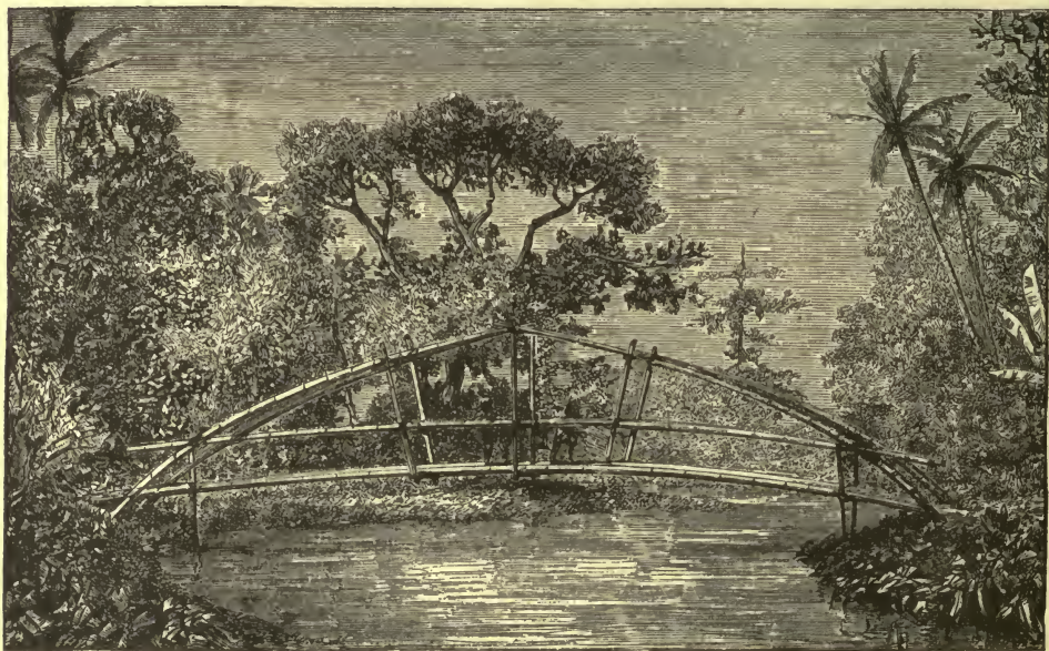
A LITTLE SUSPENSION BRIDGE OF BAMBOO.
