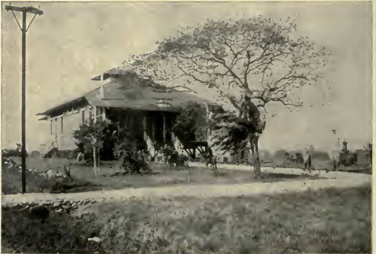
Corozal Police Station
