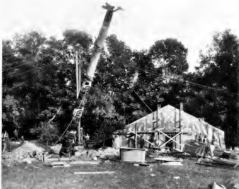
ERECTING THE TOTEM-POLE AND HOUSE.
