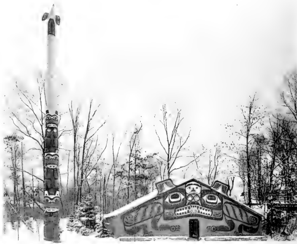
THE TOTEM-POLE AND HOUSE, AS FINISHED.
