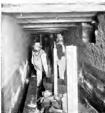
CONSTRUCTING PIPE GALLERIES.
