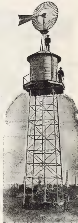
Substructure and Tank with Windmill.
