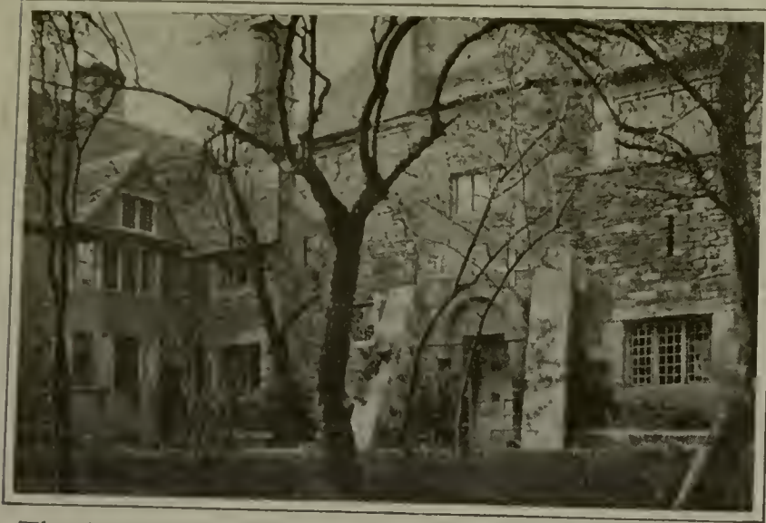
The Norman Chapel at Campden, Gloucestershire, as repaired, with additions
