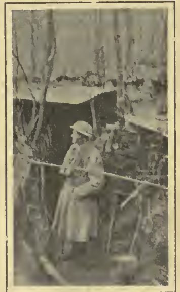
Section of Trench on American Front
