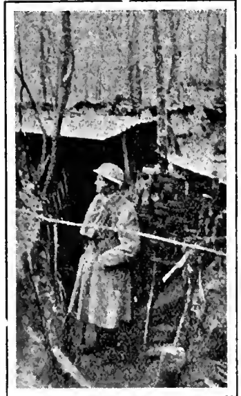
Section of Trench on American Front
