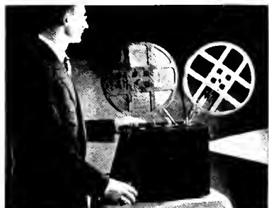
Model 33 assembles into one small compact unit. Removable top of case houses reel arms, reel and attachment cord. Speaker in baffle case is easily detached.
