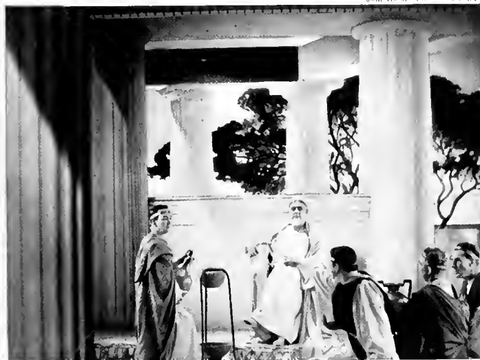
PRESTO — CHANGE-O: (BELOW) Here the camera photographs the scene with steps, properties and actors in place. The column on the extreme left was built in wood to match the columns in the projected scene. This column gave more depth to the scene. The edging of the rear-projection screen does not appear in the filmed scene.
