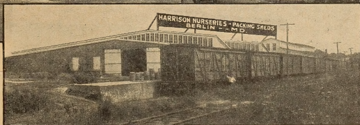
Side View of Packing Houses with Private Railway Siding Holding 35 Freight Cars
