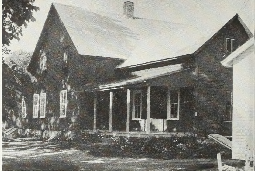
The packing house and office—just off route U.S. 7 in Charlotte.
