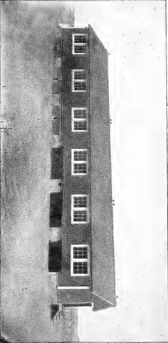
The Montana Experiment Station House. The peculiarity of this building is that the scratching sheds are underneath the laying and roosting rooms, instead of beside them, thus economizing cost of construction.
