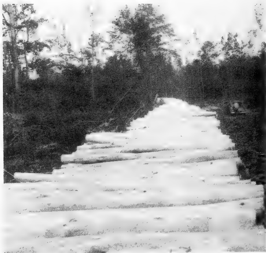
Some members of Au Sable peel their wood before shipping it to market. Compared to rough wood, peeled wood dries faster and is cheaper to haul, and pulp mills prefer it.
