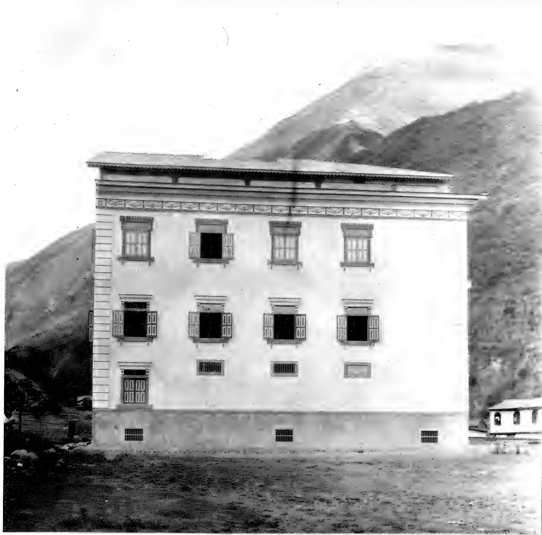
1113. A wealthy man's summer residence at Huigra (4000 feet). The walls are of two thicknesses of bamboo boards, covered with plaster or stucco.
