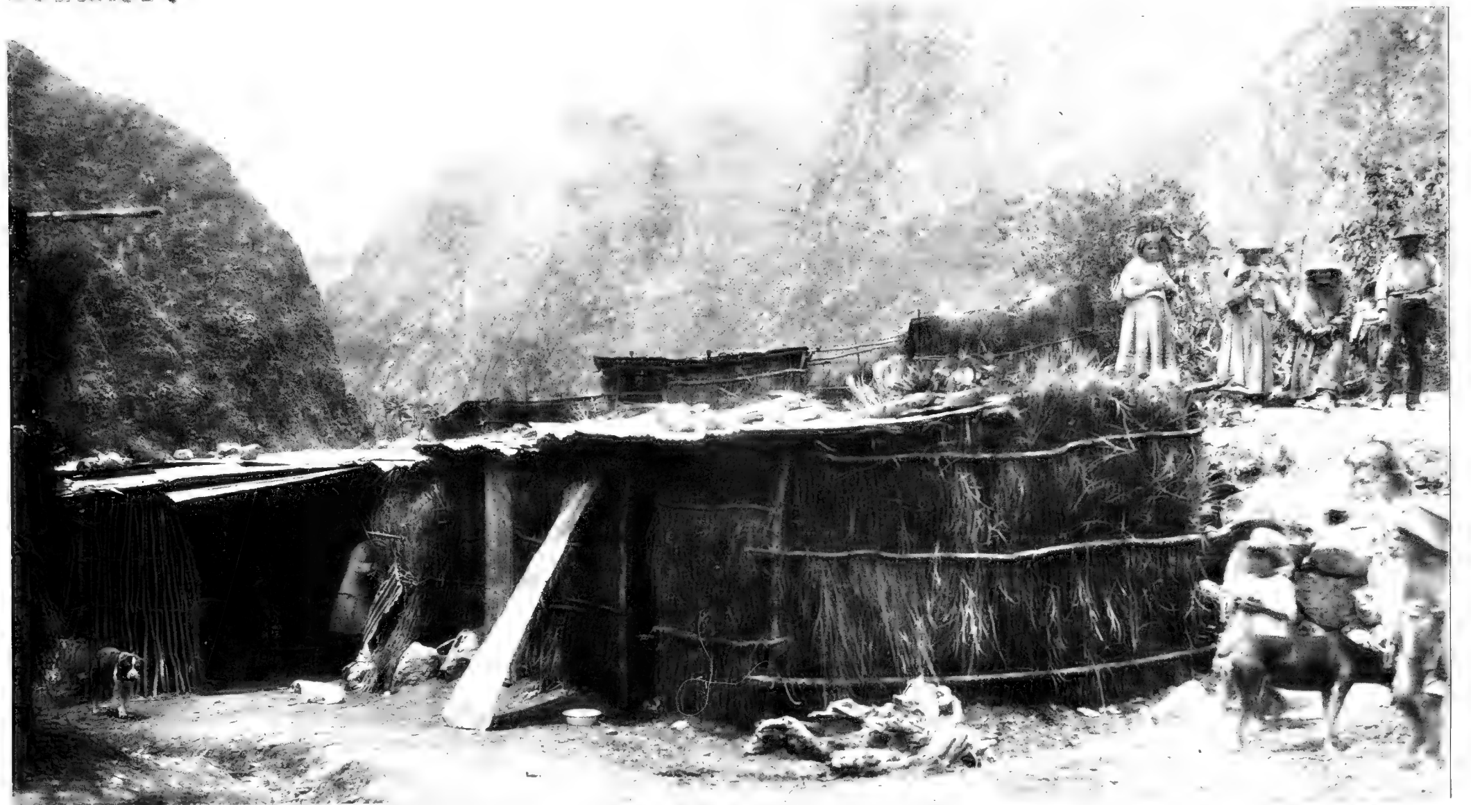
1450. A hut in the valley north of Cuzco, Peru. The sides are of brush, and the roof of corrugated iron held down with stones.
