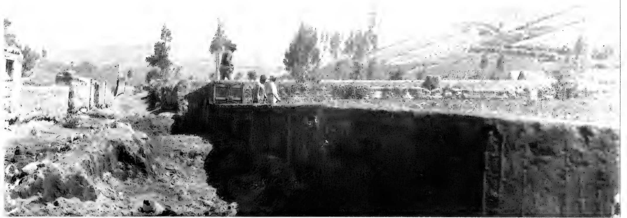
1450. A dirt wall on the uplands of Ecuador, near Ambato. The moist dirt or earth is tamped into forms of wood and hardens with age. A common method for making fences.
