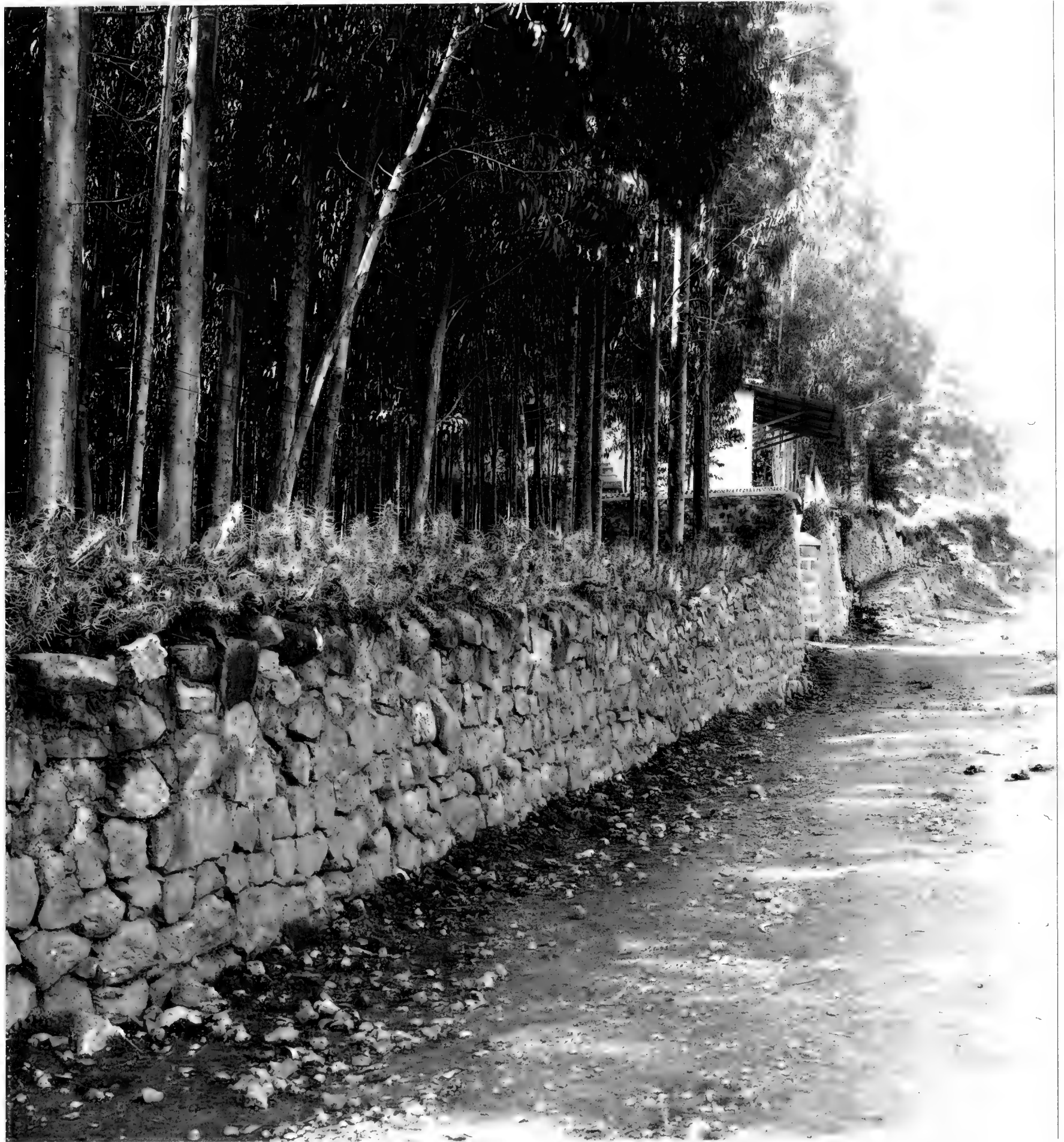
1418. A stone wall near Cuzco with cactus growing on top to prevent people from climbing over-- a common protective method. The trees are Eucalyptus.
