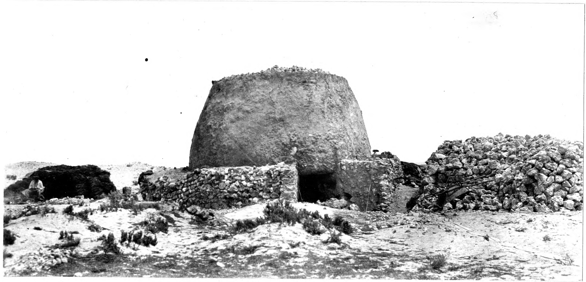
1572. A lime kiln, near Uyuni, southern Bolivia. The lime stone is in a layer at or near the surface, all over the plain. The fuel is fagots of a desert shrub obtained nearby.
