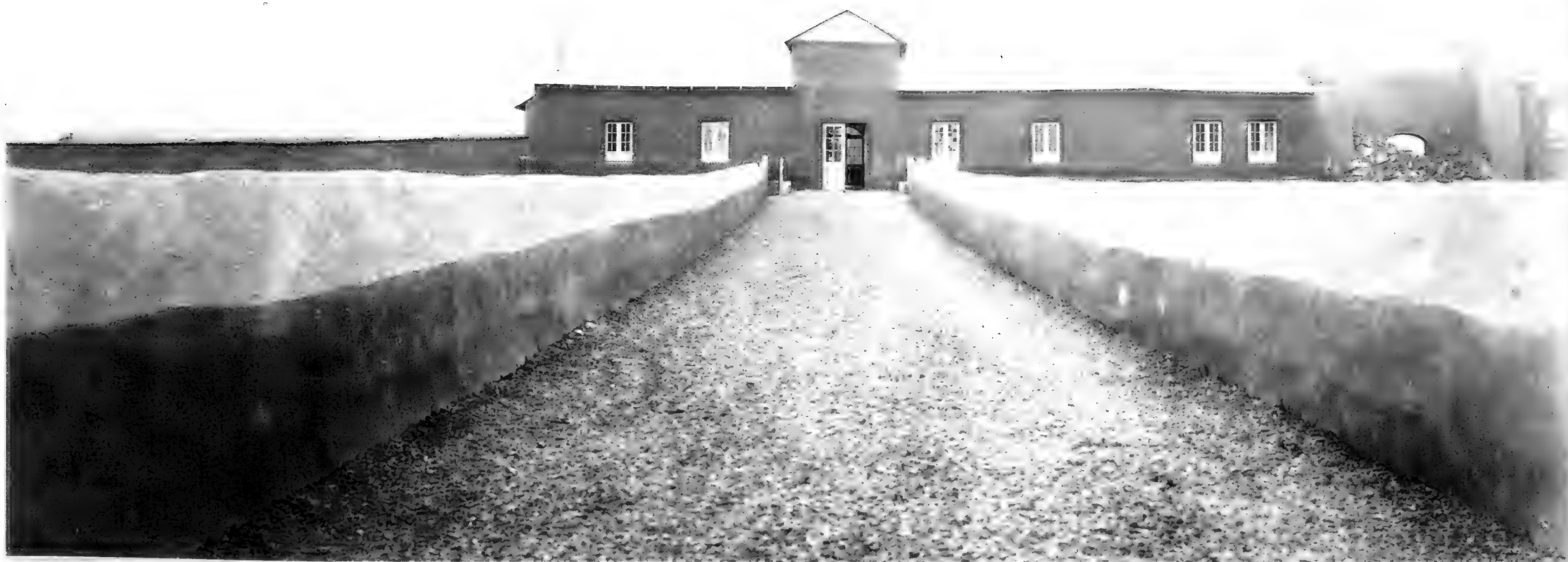
1336. The main building at the Chuquibambilla Experiment Station. The walls on either side of the road are made of adobe bricks covered with mud plaster.
