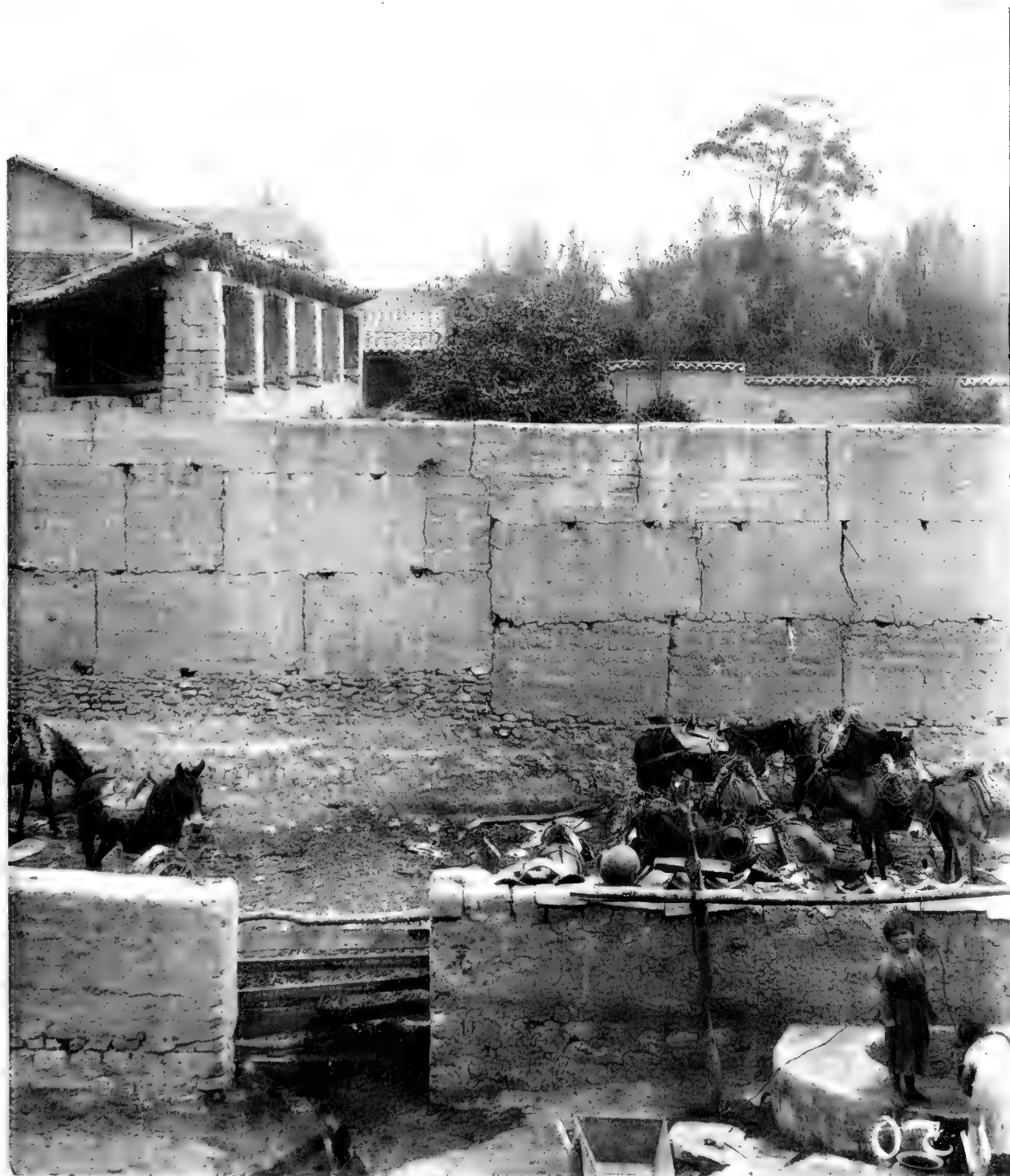
1150. The corral at the principal hotel in Loja. This was also the toilet room as there is none in the hotel building. The corral is a very filthy place. In the foreground is an open well. One needs here to boil all drinking water.
