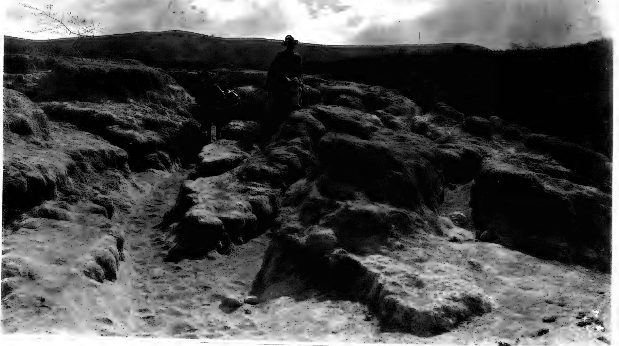
1196. A badly cut-up road in northern Cuzco pr. The main thoroughfare between Cuzco and Calcan.
