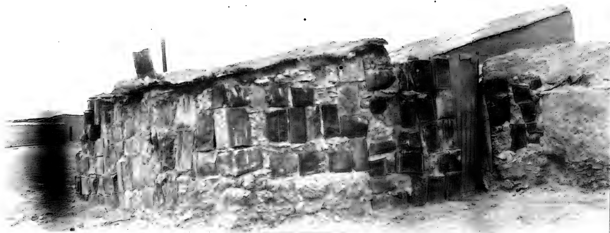
1573. A hut at Uyuni, Southern Bolivia, made of adobe and standard oil cans.
