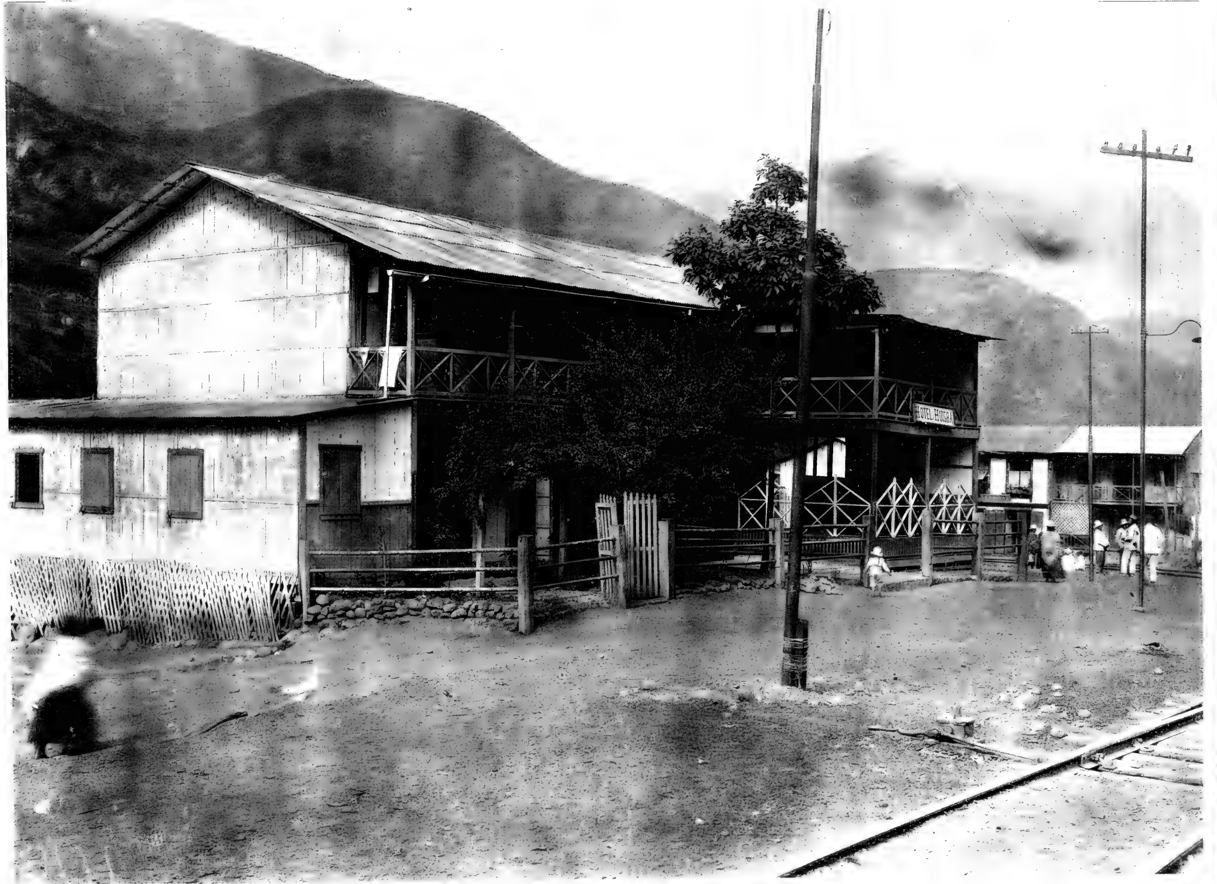
1912. The hotel at Huigra (12,000 feet) on the Huigra-Quito railroad. The walls are of split bamboo.
