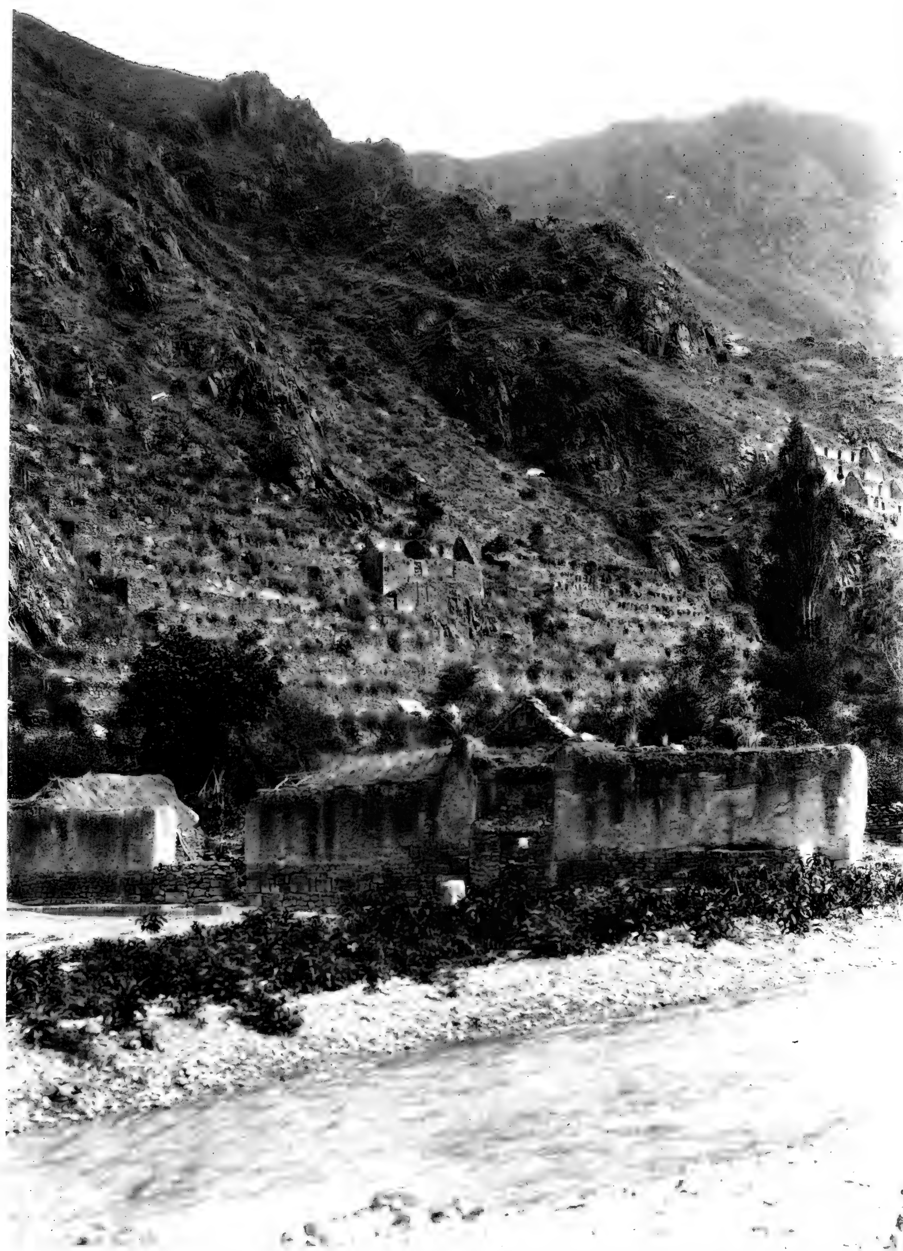
1400. Inca ruins at Ollantaytambo, Peru. On the lower part of the slope are seen a series of terraces supported by stone walls. The level ground of each terrace was used for the cultivation of crops under irrigation. The terraces are in ruins and are not now used.
