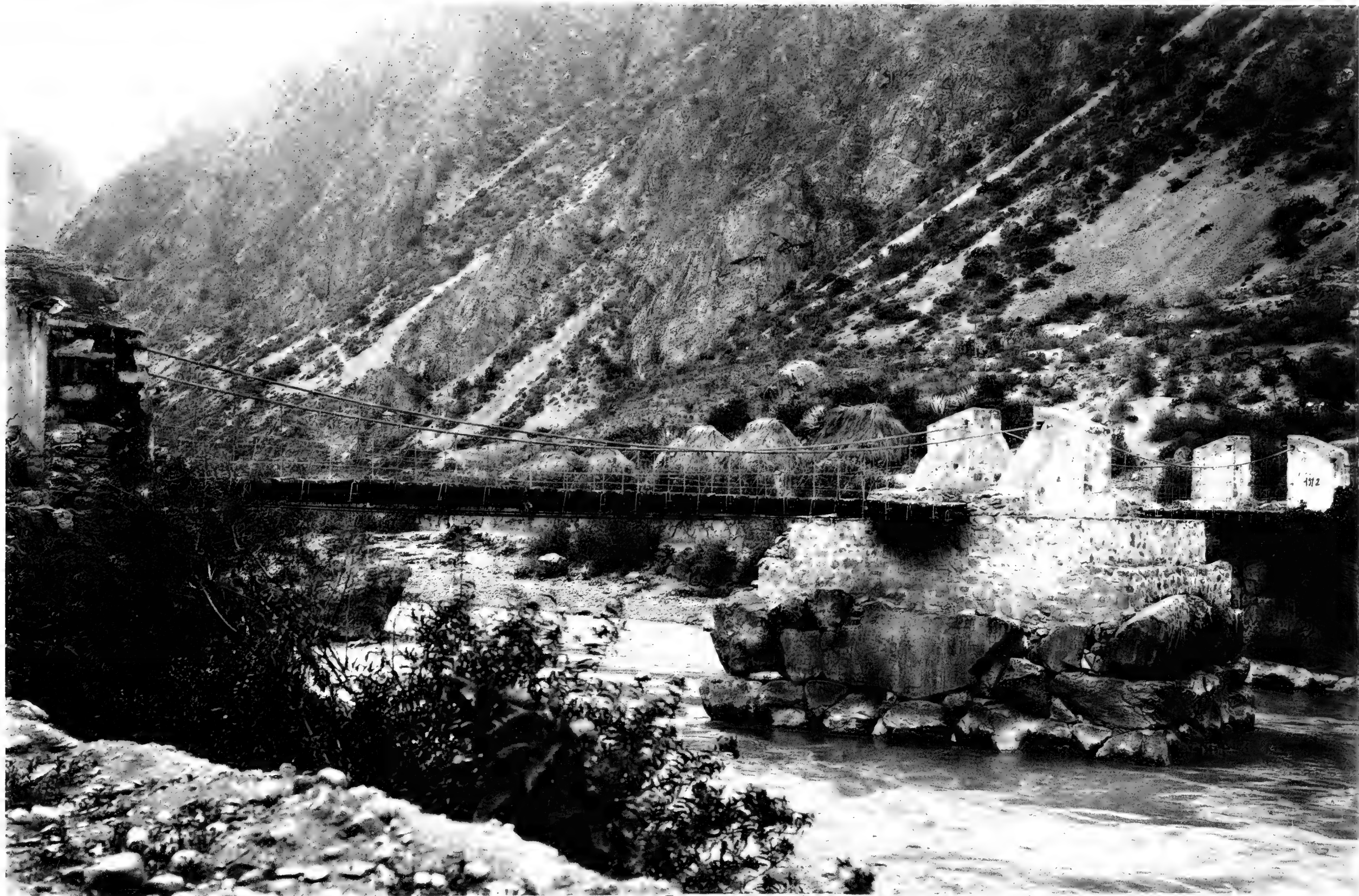
1425. Suspension bridge across the river at Tlantait, Mo., Vera. The large rocks at the base of the central pier were placed by the Incas. (Well above is cañon.)
