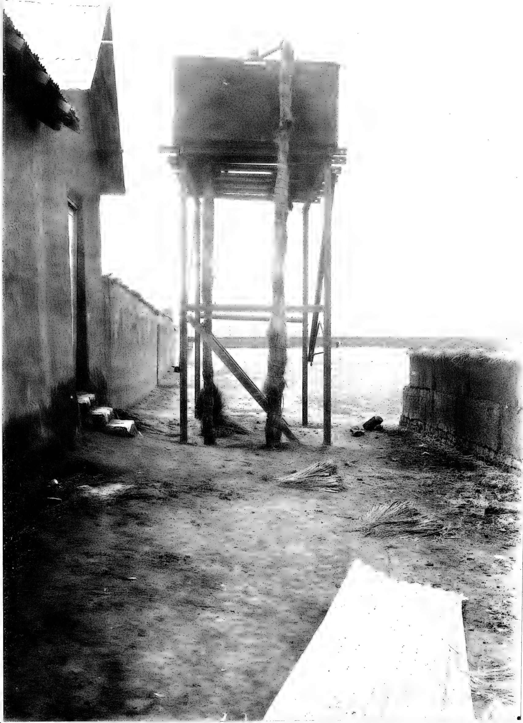
1347. A water tank at the Chuquibambilla Experiment Station. Although in the tropics, freezing temperatures are frequent, especially at night, and the pipes are wrapped with ichu grass to prevent freezing.
