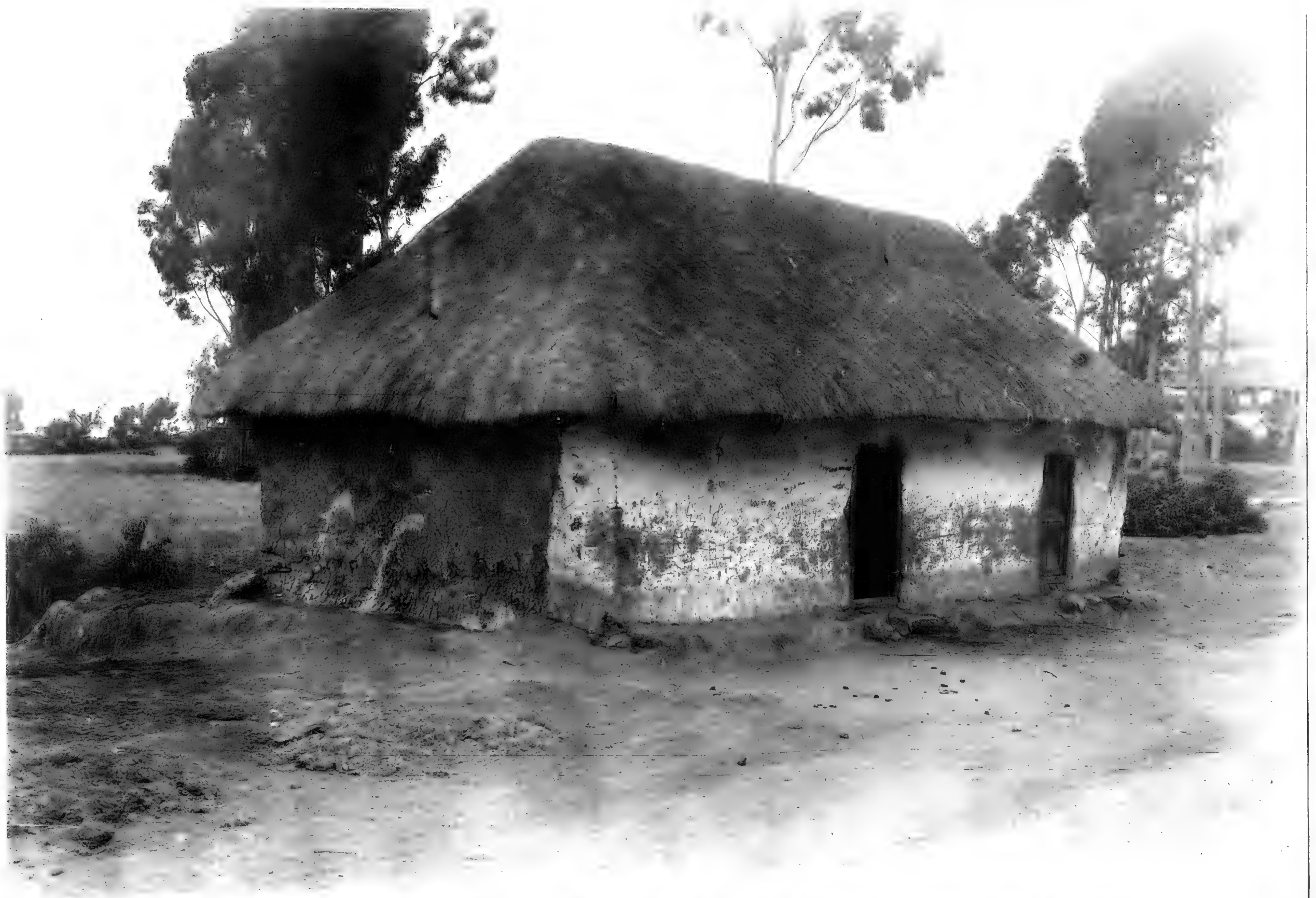
1302. Common type of hut in the uplands. The walls are of adobe bricks plastered with mud and white-washed. The roof is thatched with grass. These huts usually have no windows and no chimneys. The trees are eucalyptus, which is so only planted at 8000 to 10000 feet. It is introduced from Australia and is what we call in California blue gum. The picture taken in northern Ecuador.
