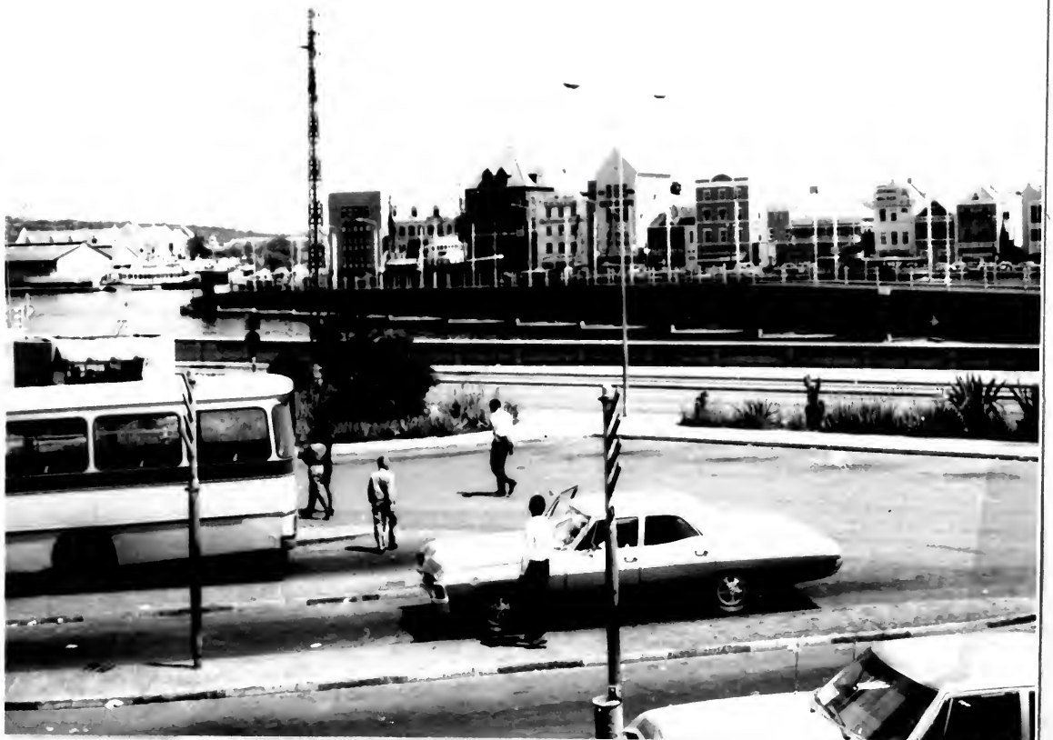
8916. The bridge swinging open to permit ship traffic. Curaçao, N.A. March 3, 1969.
