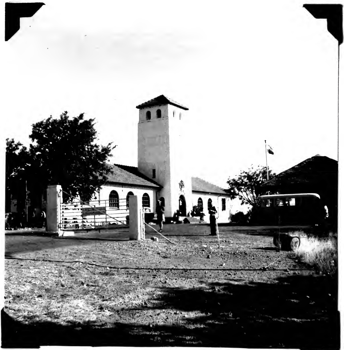
6516. Immigration and customs station for the Union of South Africa at Beit Bridge, Transvaal. July 24, 1957
