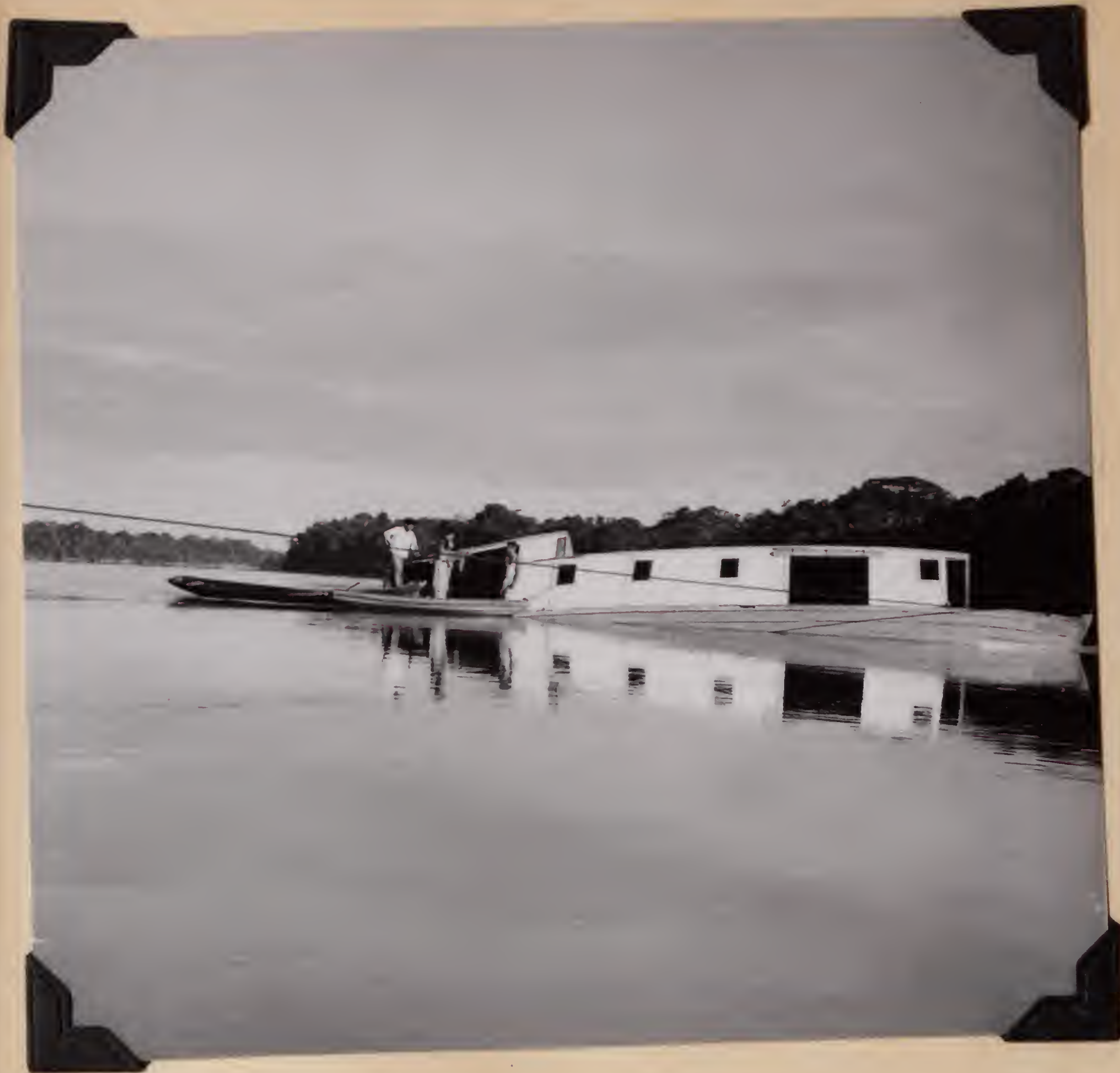
5334. The large falca sinking. Below Esperanza, Amazonas, Venezuela. January 5, 1954.
