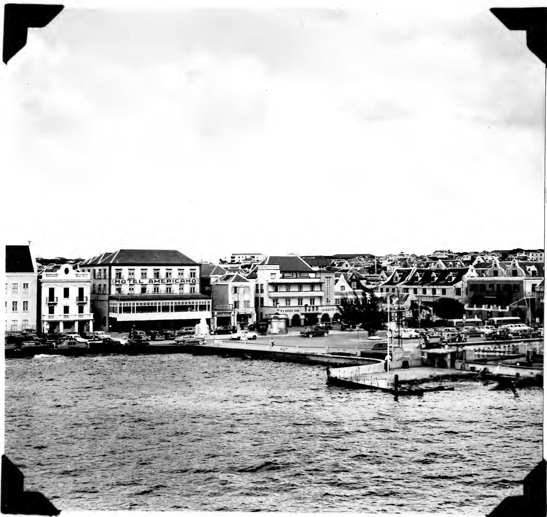
5263. Approach to bridge on Otrabanda side, Willemstad, Cura- çao. December 21, 1953.
