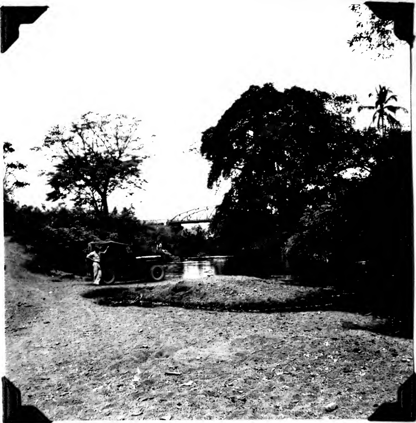
3599. Bridge on the Río Las Tablas, near Guararé, Los Santos. March 28, 1948.
