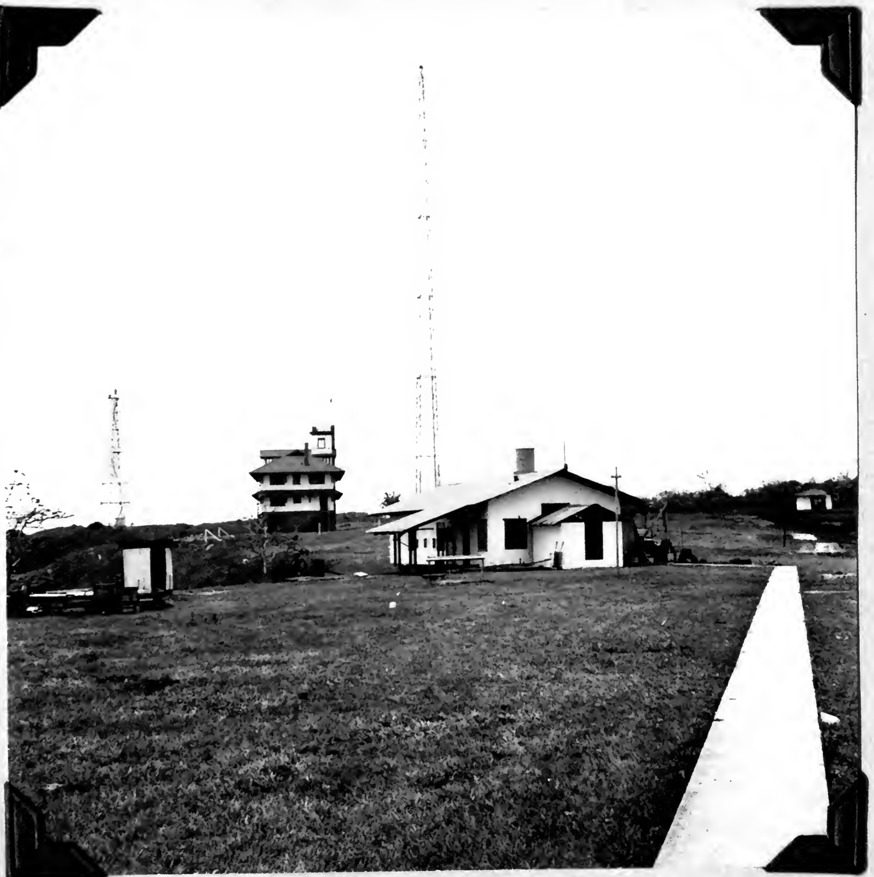
3572. Light house, living quarters, radio beacon and generator house at Punta Mala, Los Santos. March 27, 1948.
