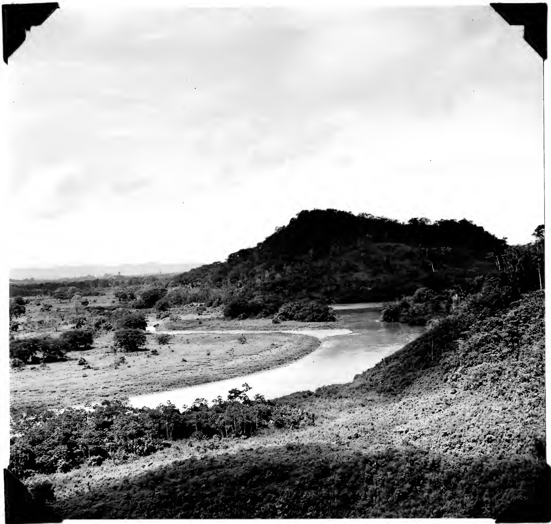
5168. A branch of Río Tabasará, near the road bridge. Taken from near Quebrada Piedra, Chiriquí. June 6, 1953.
