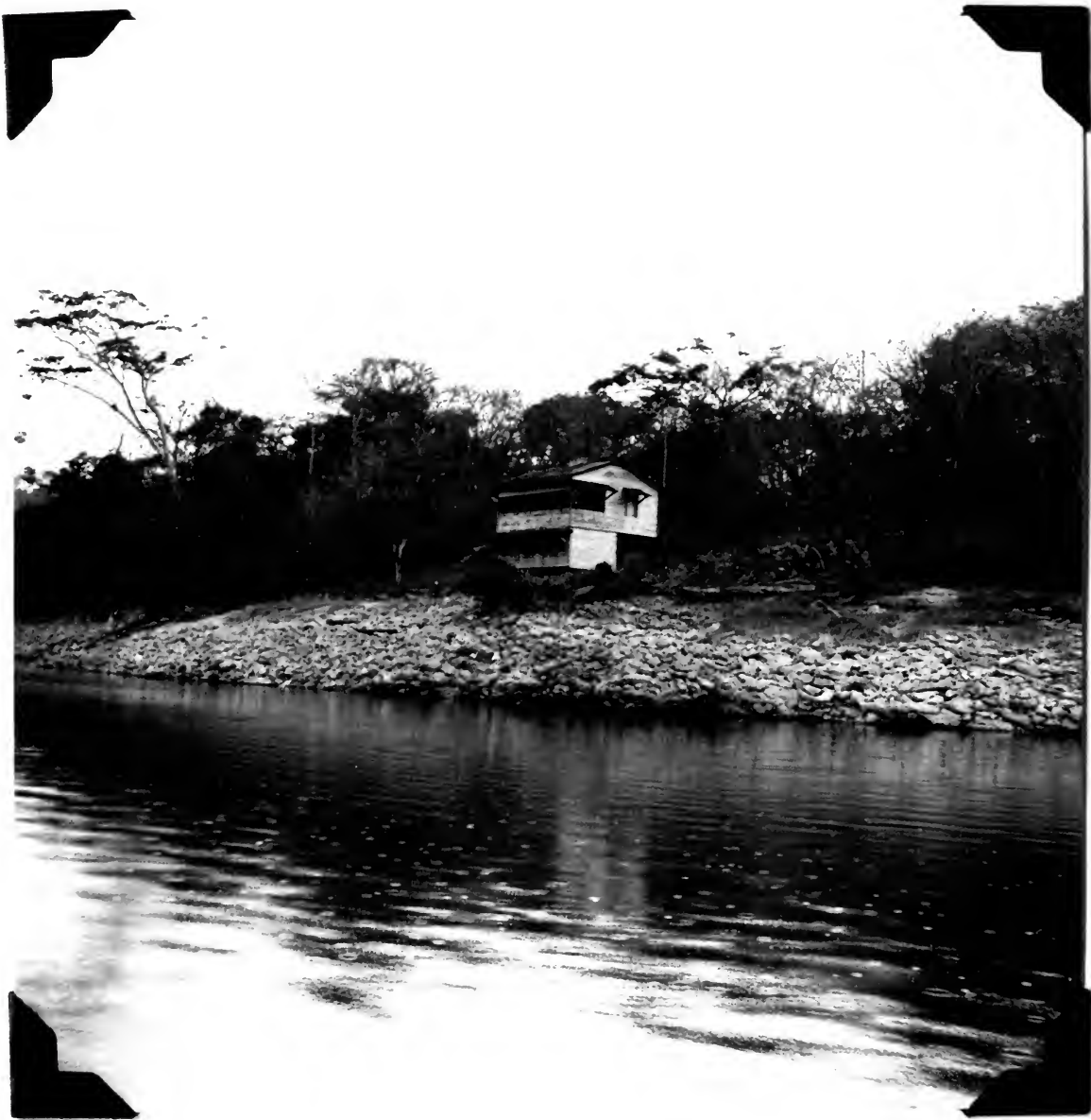
8317. Salamanca Hydro- graphic Station on Madden Lake, now abandoned, where Griswold worked in 1936. March 13, 1961.
