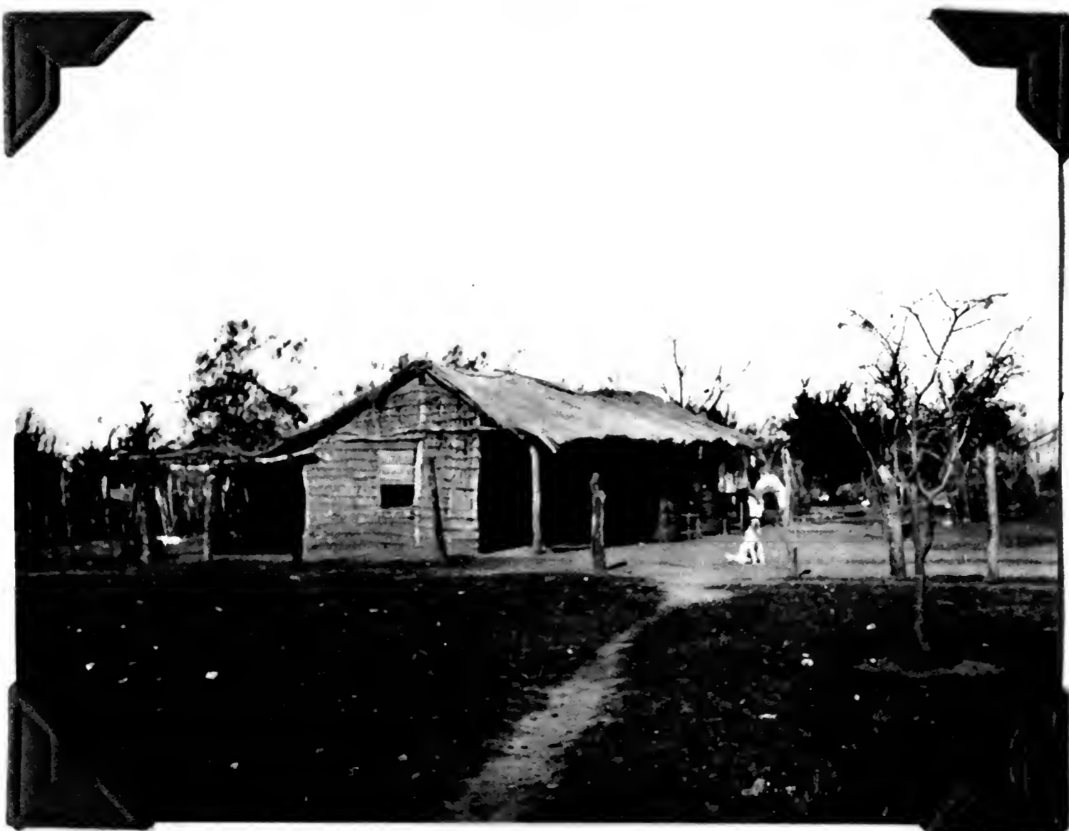
B.S. 21968. A grass-thatched hut built of mud plastered on a frame of wood. Las Palmas, Chaco Argentina. July 19, 1920.
