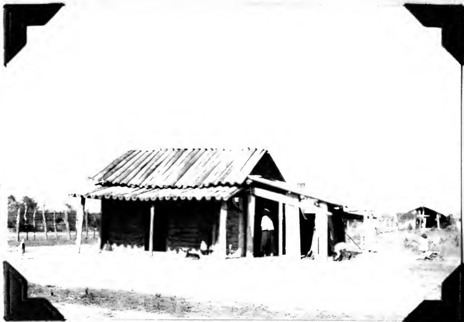
1353. House with roof of split palm trunks. Las Palmas, Chaco, Argentina. July 19, 1920.
