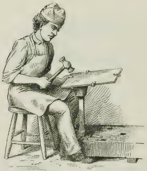
Fig. 19.—Planishing at the Block.
